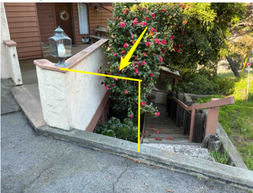
Location of a recommended railing
