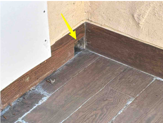
A single scupper drain
