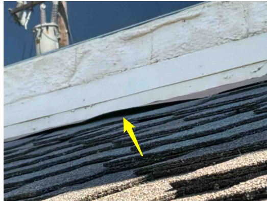
Example. At some head wall flash
