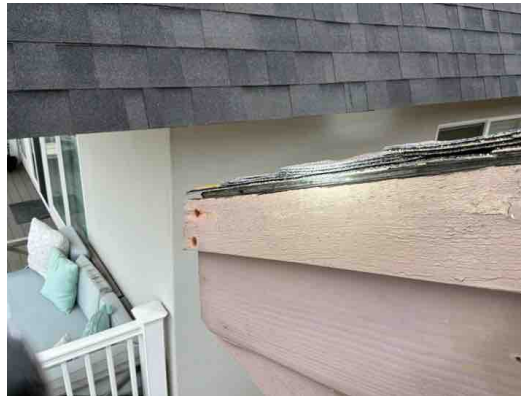
Exposed roof plywood
