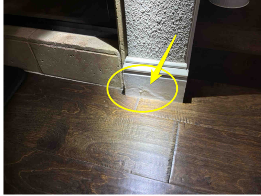
FI 164: Some minor moisture stains and swelling of the baseboards at the walls outside shower: DOWNSTAIRS PRIMARY BEDROOM BATHROOM
