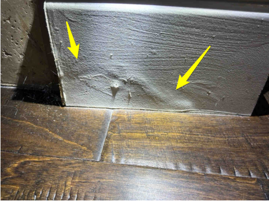
FI 164: Some minor moisture stains and swelling of the baseboards at the walls outside shower: DOWNSTAIRS PRIMARY BEDROOM BATHROOM
