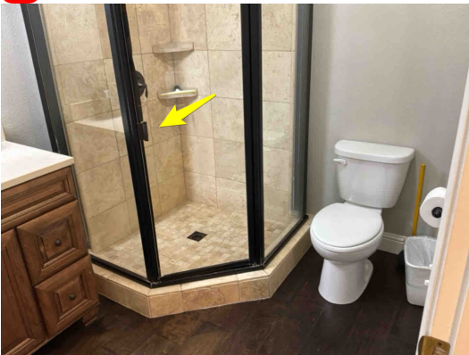
E&C 165: Glass shower door does not seal or latch well: UPSTAIRS HALL
