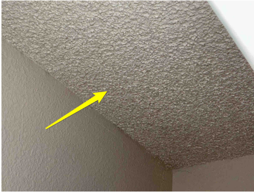
Example. Inside a closet
