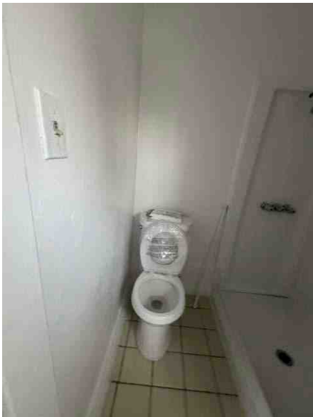
UNIT A-Bathroom Pic 1 of 2
