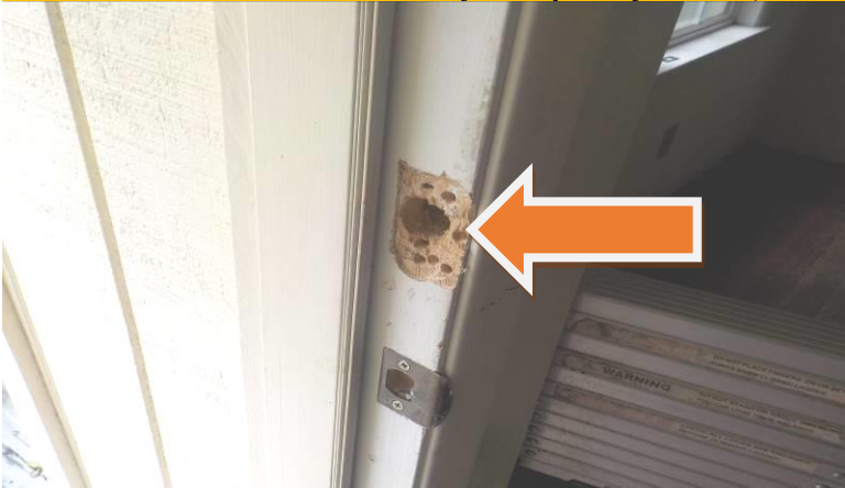
Item #18-Fascia-At the west end of the home, wood damage to the fascia board behind the rain gutter
