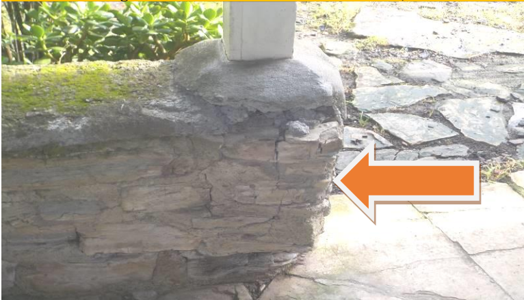
Item #6-Steps-At the rear deck, I recommend adding a maximum 2" diameter 'grab rail' to the top or side of the 2x6 rail cap
