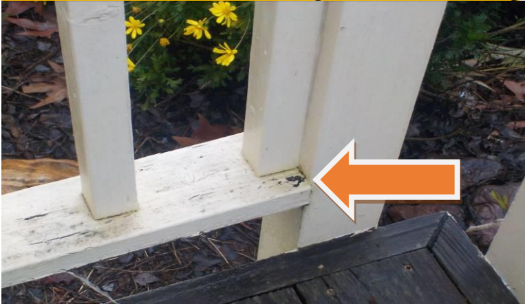
Item #15-Exterior doors-At the rear entry to the primary bedroom, the deadbolt strike plate on the door frame is missing/damaging the frame
