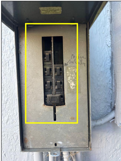
Main electrical service panel to the home.
