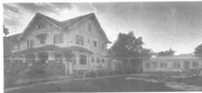
1988 photo of a large home on Oxford Avenue undergoing restoration.
