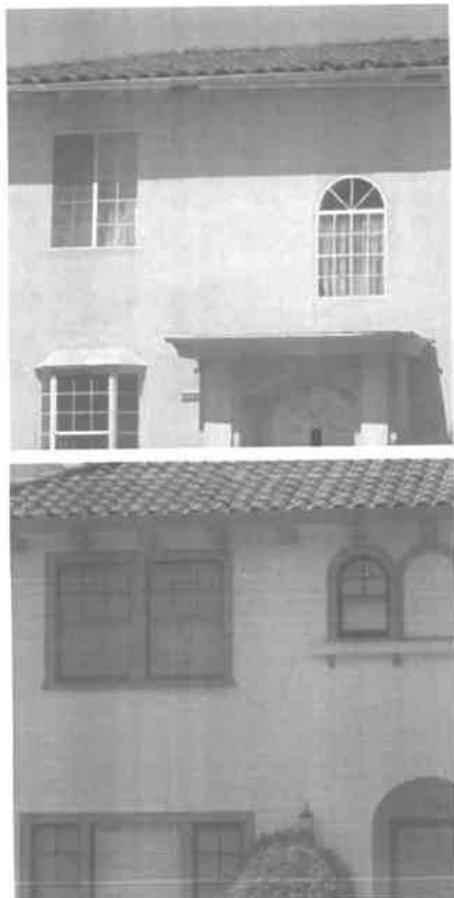
Flush, frameless, and oddly arranged windows may be inappropriate on a new house.
