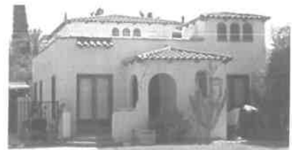
This second-story addition is set-back and preserves the look and scale of the original bungalow.
