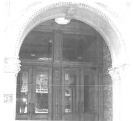
Attention should be paid to the materials and decorative features of a building entrance.
