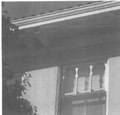
Smooth, hand-trowled stucco is an appropriate finish for this Italian Renaissance Revival home.
