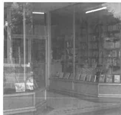
Bulkheads allow for storefront displays as well as the placement of durable and decorative materials along the storefront.
