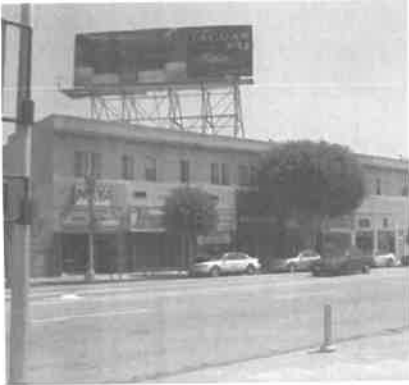
Storefront improvements should be consistent with the overall building facade. This building has been chopped into irreconcilable pieces.
