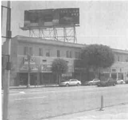
Storefront improvements should be consistent with the overall building facade. This building has been chopped into irreconcilable pieces.
