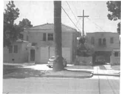
Many historic neighborhoods were built with accessory living quarters over garages. Attention should be paid to the historic precedent on your street.
