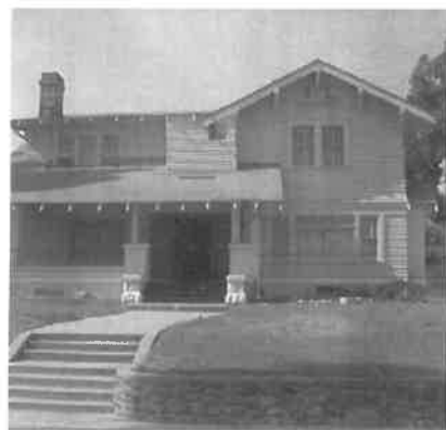
Historic retaining walls often comprised of stone are an important part of the neighborhood setting.
