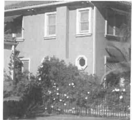
Foam plant-ons and pre-cast concrete are materials that would not have been originally used on this historic house.
