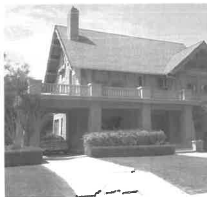
The porch, porte-cochere and balcony are a prominent feature on this Tudor-Craftsman house.
