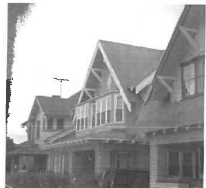
This street presents a consistent roof pattern that should be replicated on new construction.
