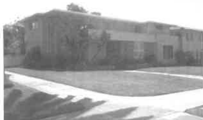
Houses of varying styles and periods may co-exist harmoniously by virtue of their similar massing and orientation.
