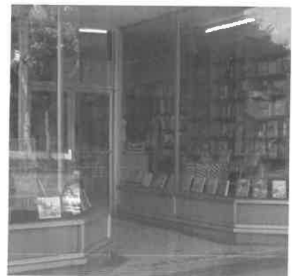
Bulkheads allow for storefront displays as well as the placement of durable and decorative materials along the storefront.
