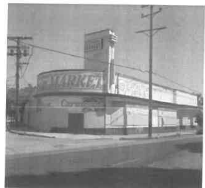
Doors and windows have been removed from this building (in favor of a rear-facing parking lot), to the detriment of the street.
