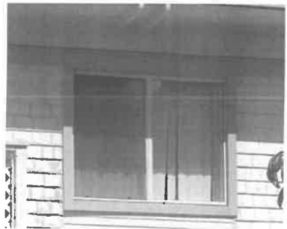
An inappropriately sized aluminum window diminishes the historic value of a house.
