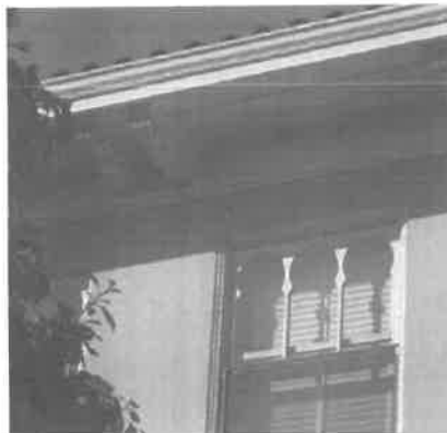
Smooth, hand-trowled stucco is an appropriate finish for this Italian Renaissance Revival home.
