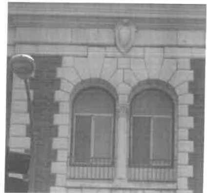
Pilasters, quoins and lintels are used on this building facade.
