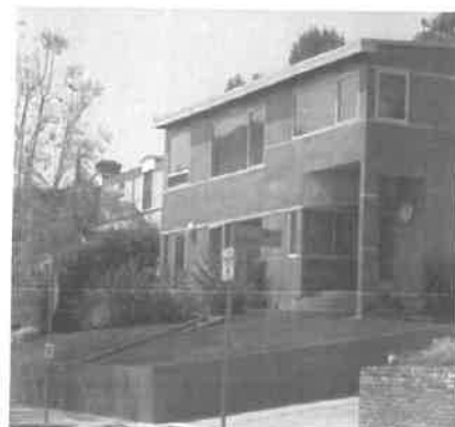
Though innovative and interesting, the materials on this home do not relate to those used in its surroundings.
