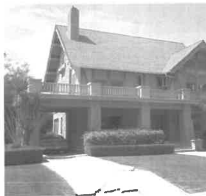
The porch, porte-cochere and balcony are a prominent feature on this Tudor-Craftsman house.
