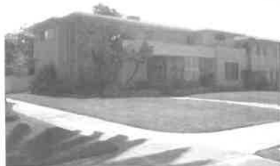
Houses of varying styles and periods may co-exist harmoniously by virtue of their similar massing and orientation.
