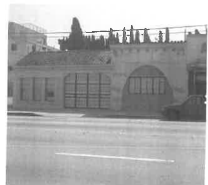
Concrete block is not a material that is original to this Spanish Colonial building.
