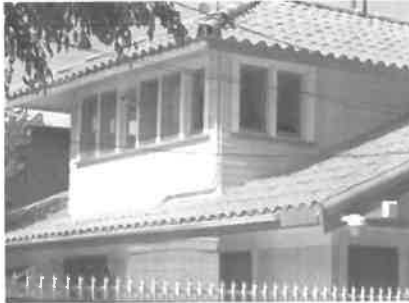
Clay tile is an inappropriate material for this Craftsman style home.
