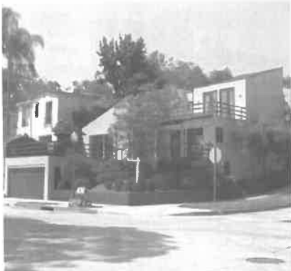
Though different in style, this house's deep, and vertical openings help it to blend with its neighbors.
