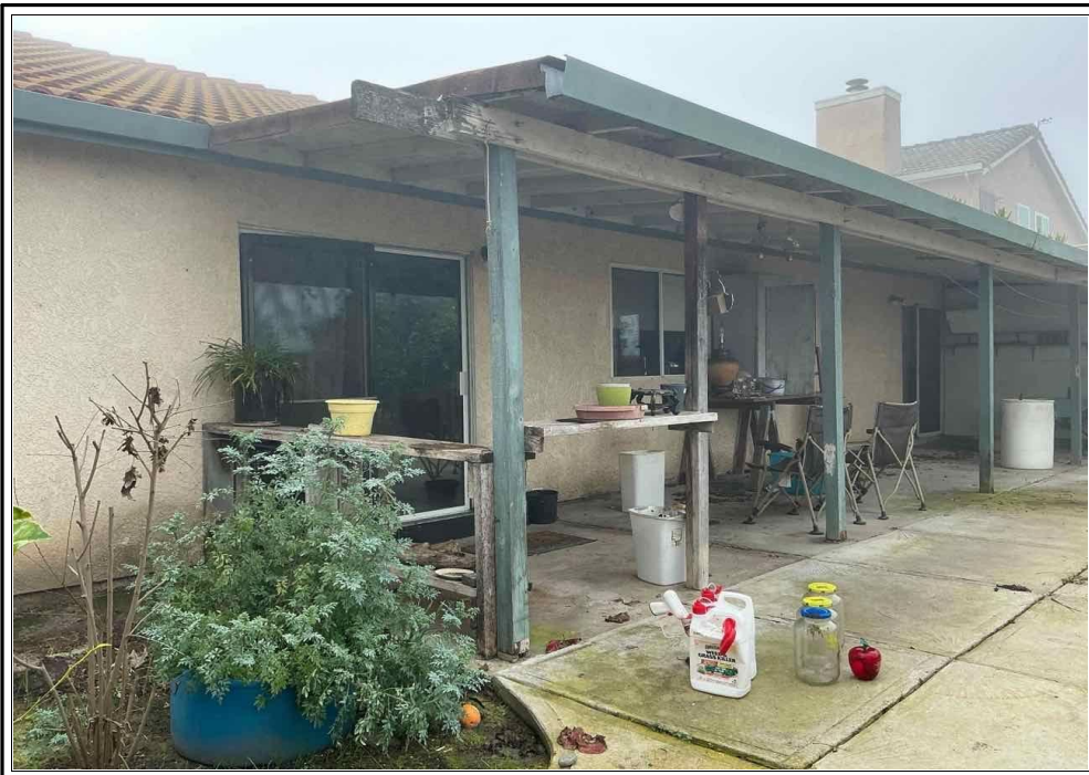
REAR OF SUBJECT PROPERTY
