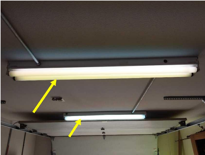
A light is missing its globe or cover and should be serviced.
