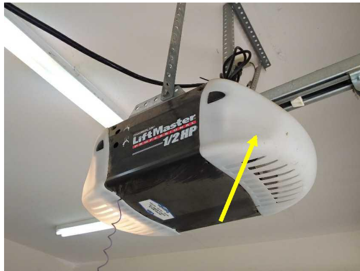
The garage door opener front light did not respond when the auto-reverse mechanism when activated which should be serviced. This is important because it typically is the only light on when pulling into the garage at night.
