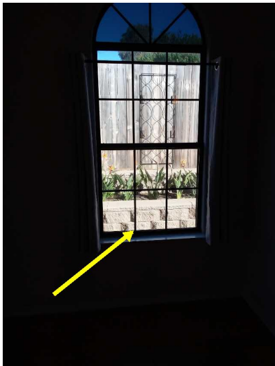
A window is stuck or painted shut, and should be serviced.
