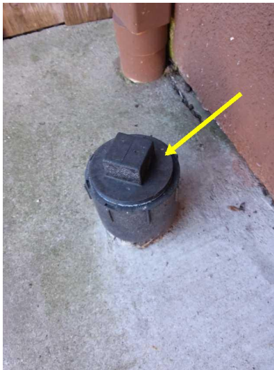
A clean-out is located at the rear.
