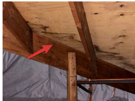
Under roof valley
