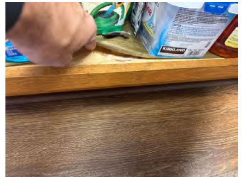
Base of kitchen sink cabinet
