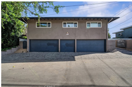
Six garage spaces
