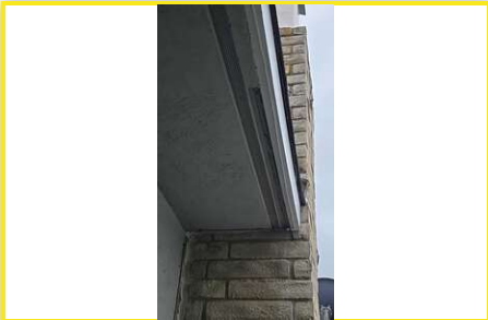
Location: WEST SOFFIT
