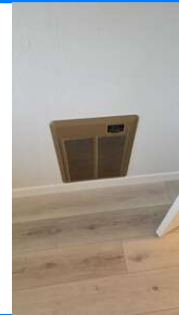
Location: FRONT BEDROOM
