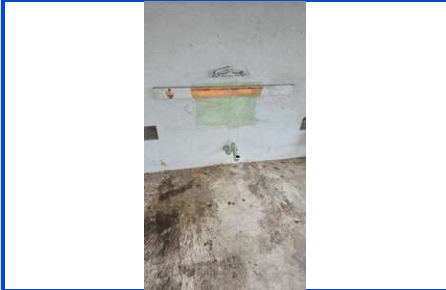
Location: NORTH EXTERIOR
