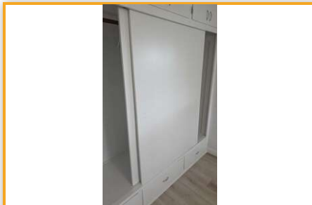
Location: FRONT BEDROOM
