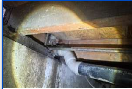
Location: KITCHEN CRAWLSPACE
