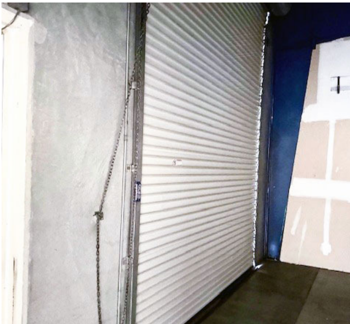
Ste 1/2 - 2nd Warehouse section and 2nd Rollup Door
