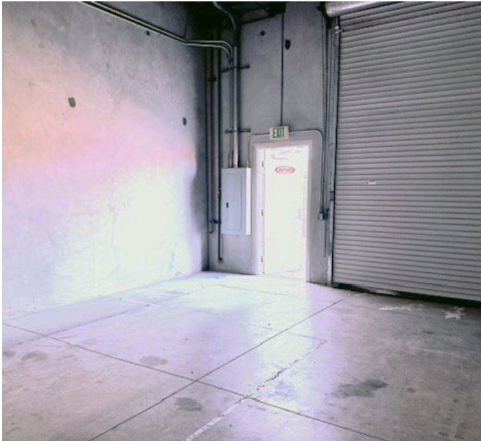
Ste 1/2 - Warehouse with Roll Up and Door
