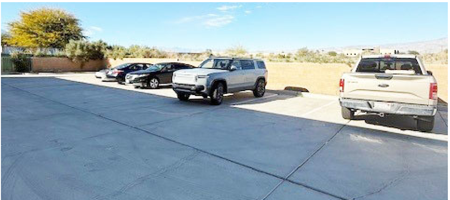
Ste 4/5 - Rear parking lot
