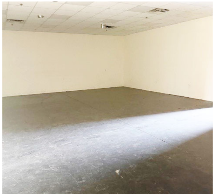
Ste 4/5 - Middle Area with Restroom Access
