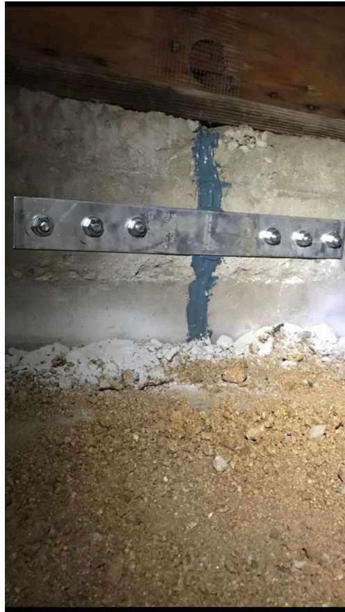
Epoxy and Simpson HST-2 strap (sample photo)
