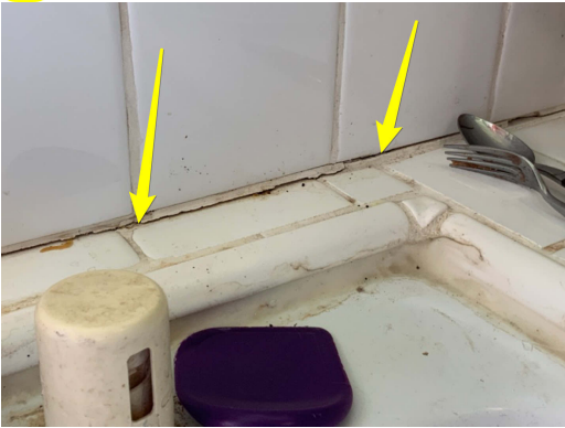
This can allow water to flow into the cabinetry below
