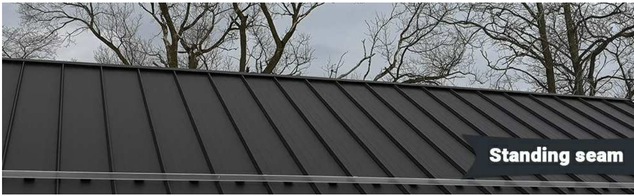
11 STANDING SEAM METAL ROOF
