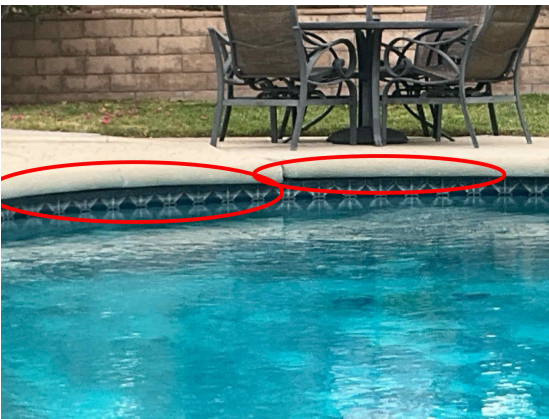
Lifting concrete
