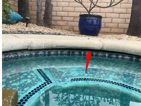
Lifting concrete
