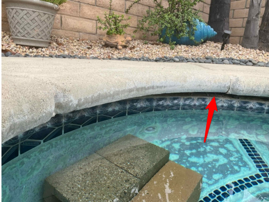
Lifting concrete
