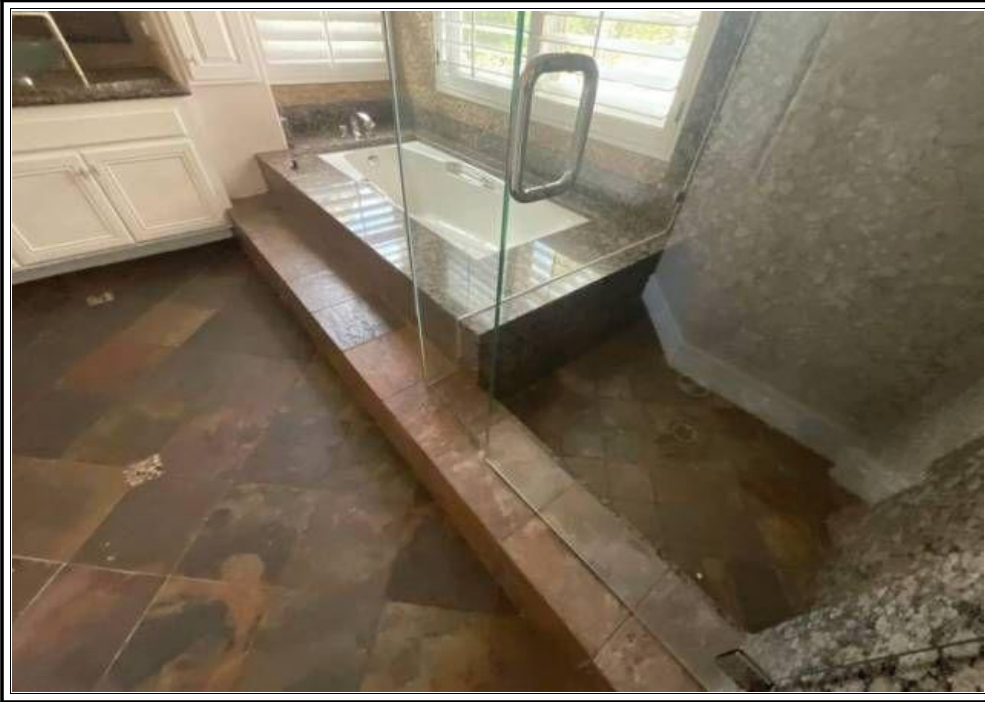
BATHROOM 3 GLASS SHOWER DOORS / TILE SHOWER
