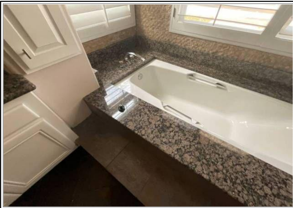
BATHROOM 3 BATHROOM TUB
