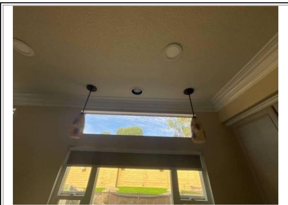
KITCHEN LIGHT FIXTURES
