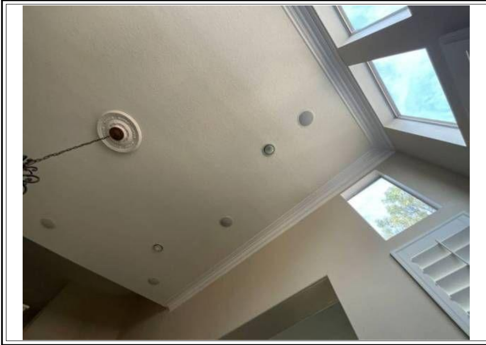
RECESSED LIGHTING BUILT IN SPEAKER
