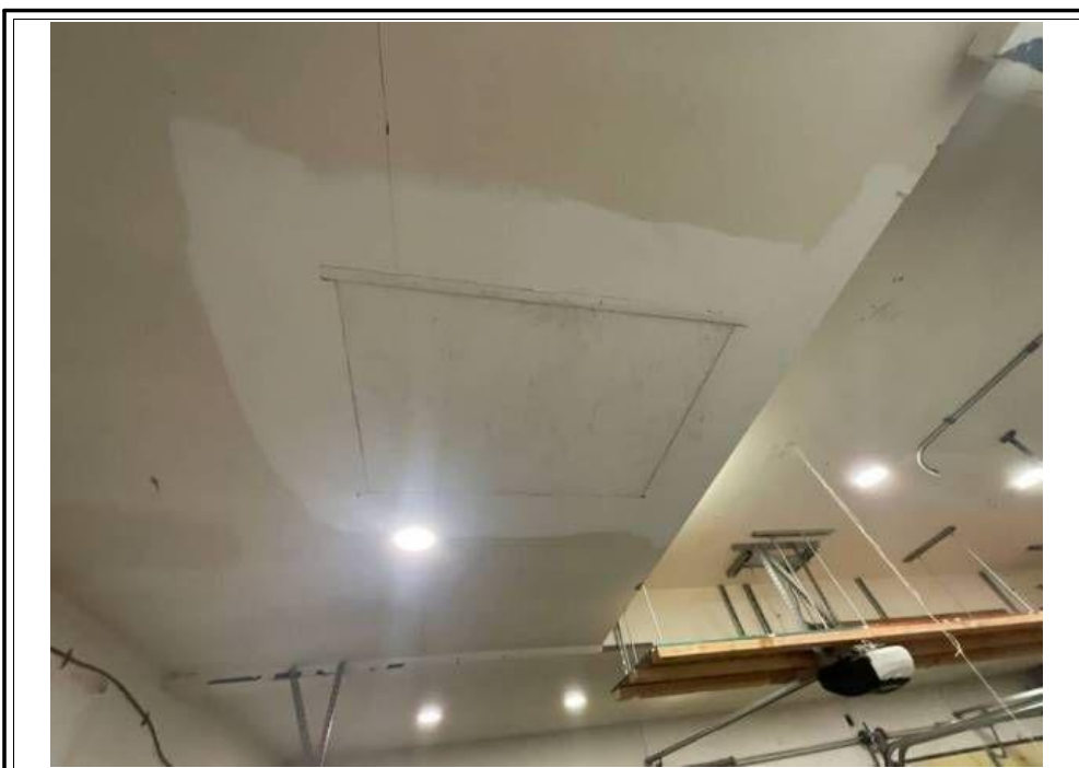
GARAGE ATTIC ACCESS
