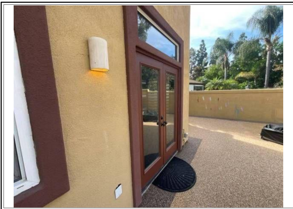
REAR ENTRY DOOR
