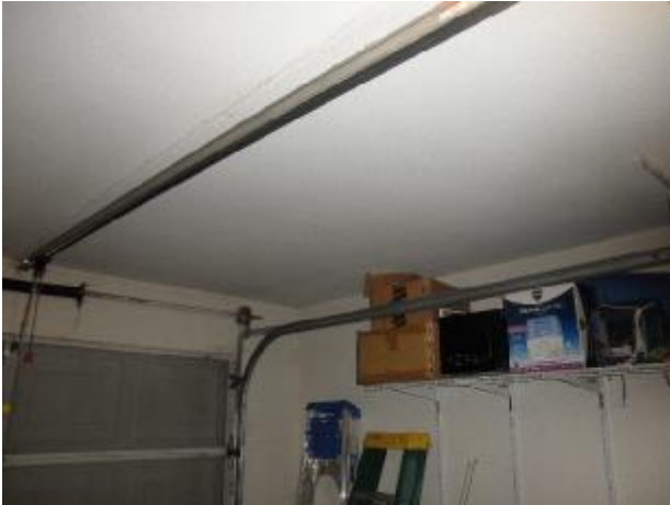
No leaks observed below the water proof deck.
