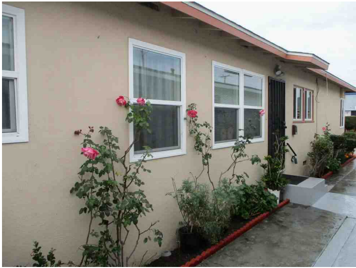
FRONT OF UNIT 2
