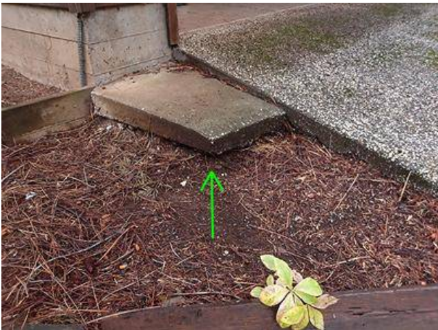
Photo 9-1 NE corner garage
