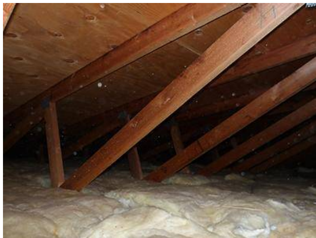
Photo 21-4 Attic insulation above sloped ceiling
