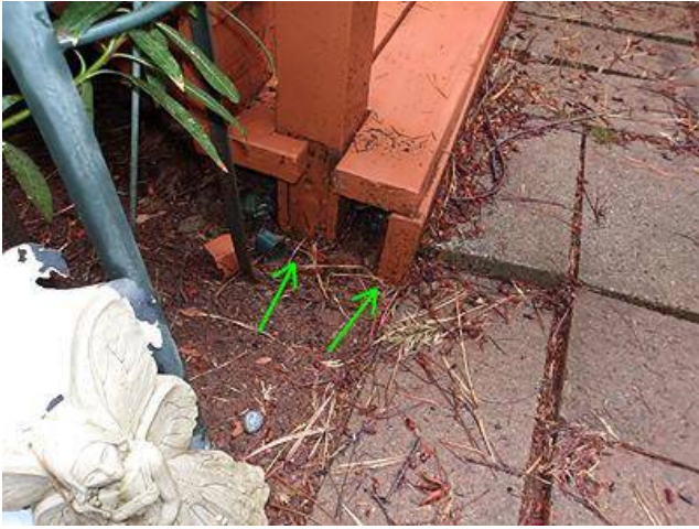
Photo 8-3 West deck stairs
