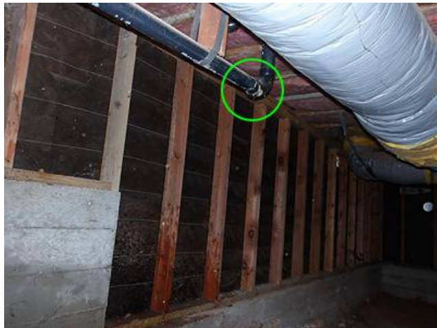
Photo 48-2 Master bathtub drain line
