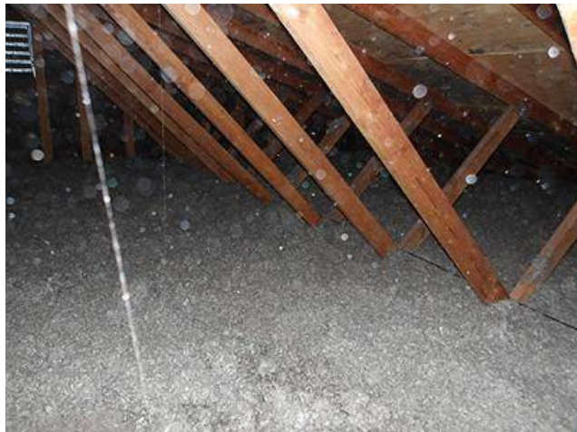
Photo 21-2 Attic insulation
