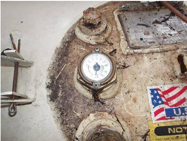
Photo 55-1 Propane tank empty
