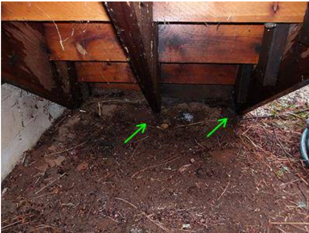
Photo 8-1 Front porch stairs
