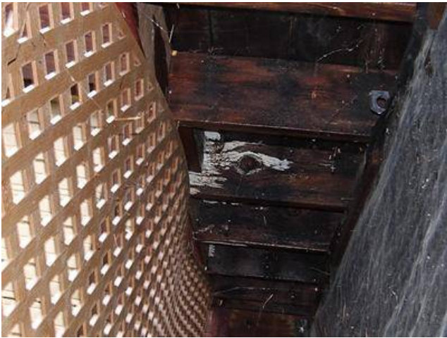
Photo 5-1 Front porch joists
