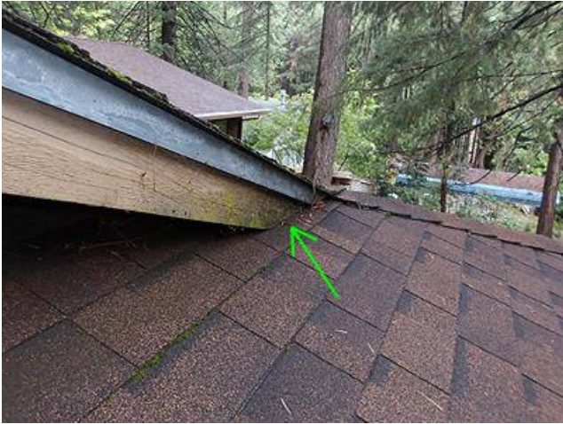
Photo 24-1 NE corner garage
