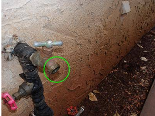
Photo 51-2 SW corner garage
