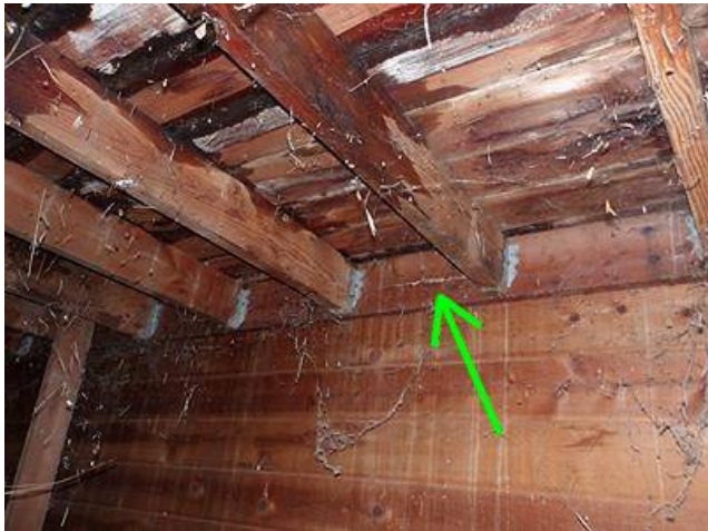
Photo 3-1 Front porch ledger board
