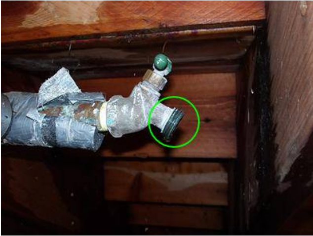
Photo 51-1 East side below stairs
