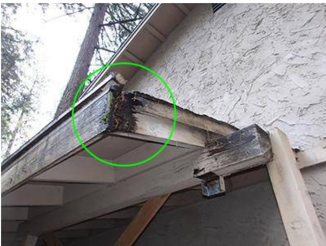
Photo 17-1 North side above HVAC unit
