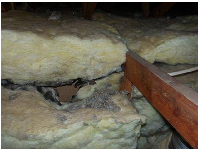
Photo 21-3 Attic insulation above sloped ceiling
