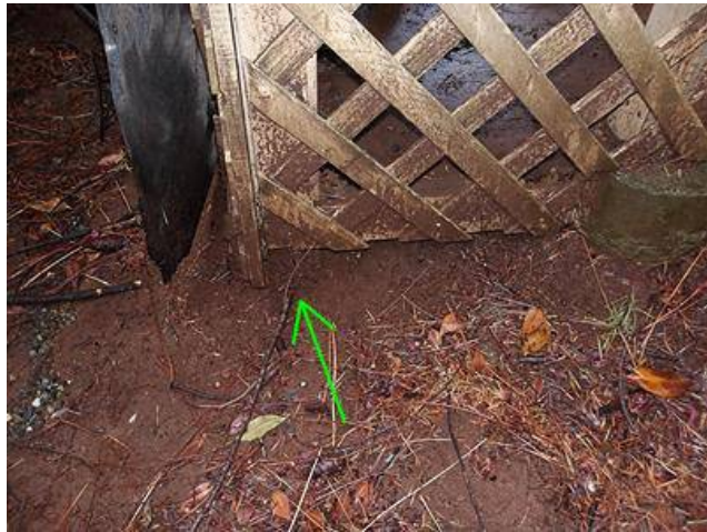
Photo 8-2 NW corner carport
