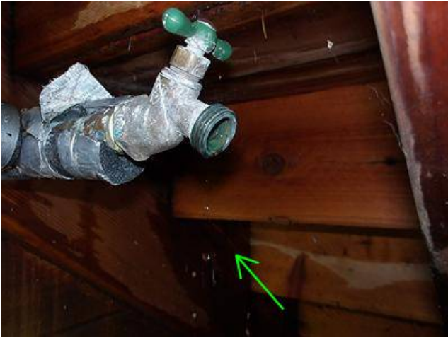
Photo 50-1 East side below stairs
