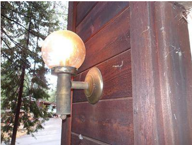
Photo 42-3 NE corner garage
