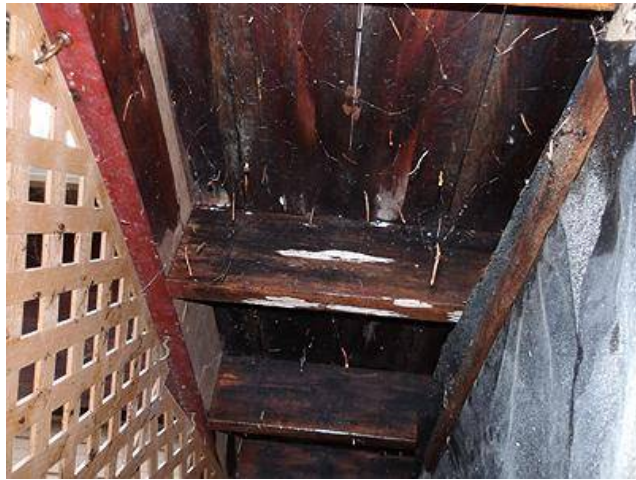
Photo 5-2 Front porch joist
