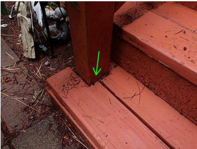
Photo 6-3 West deck stairs
