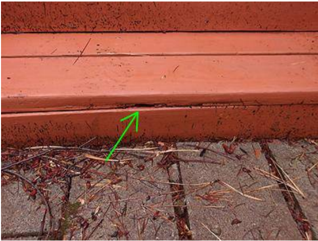
Photo 6-1 West deck stairs
