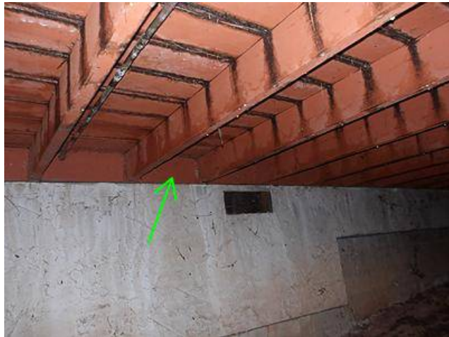
Photo 3-2 West deck ledger board
