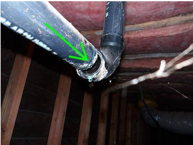
Photo 48-1 Master bathtub drain line
