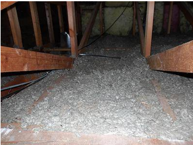
Photo 21-1 Attic insulation
