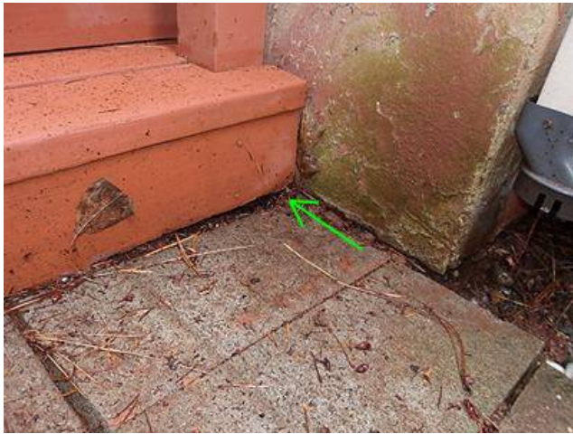
Photo 6-2 West deck stairs
