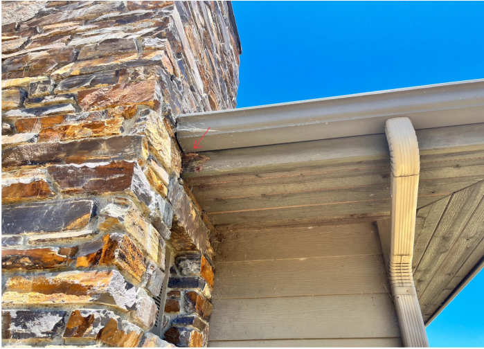
3A - Damage to the fascia board
