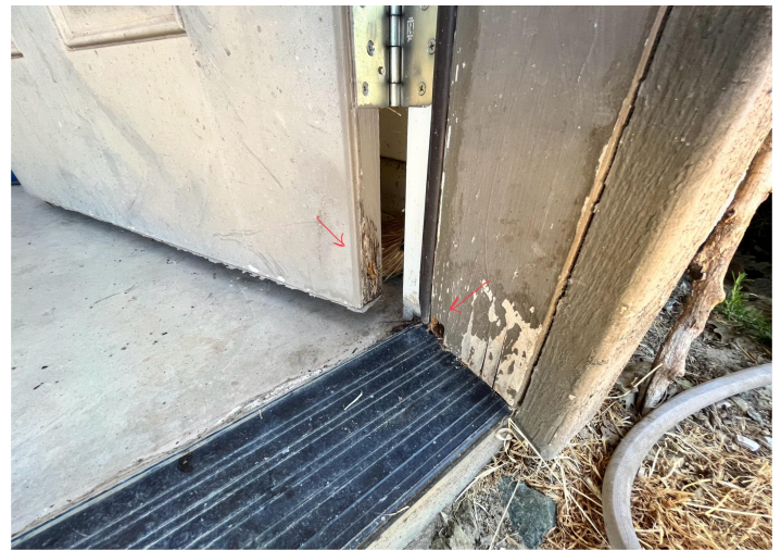
3A & 3B Example of damage to the fascia and patio framing.
