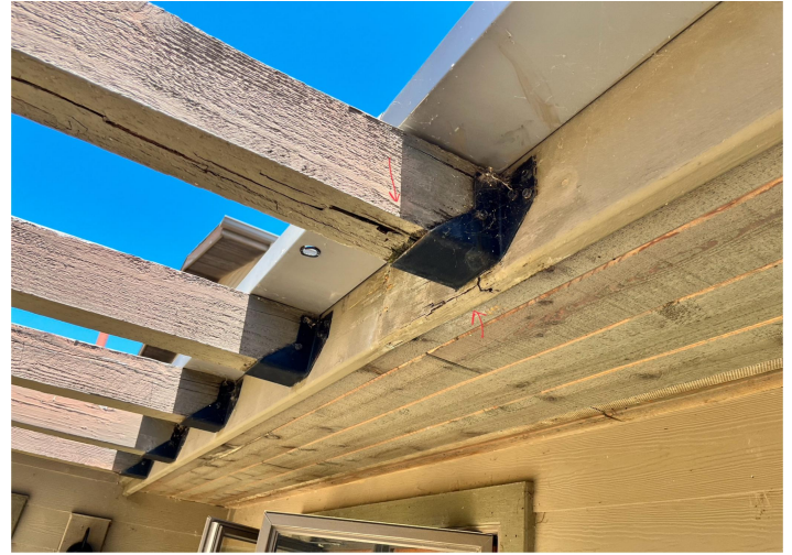
3A & 3B Example of damage to the fascia and patio framing.
