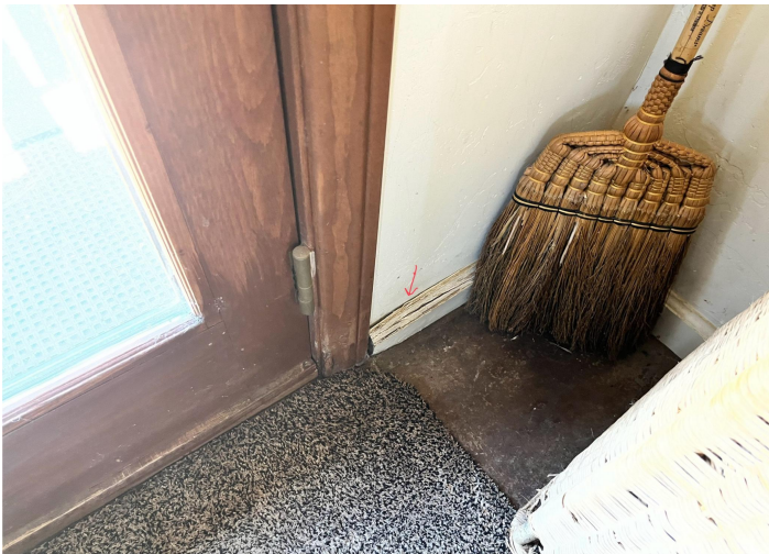
3C - Damage to laundry room door
