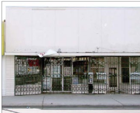
Unacceptable security bars.
