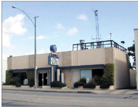
Exposed roof-mounted equipment is prohibited.
