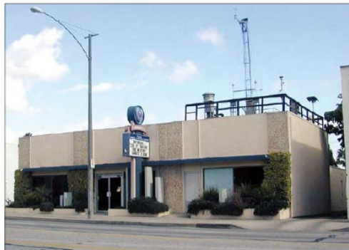
Exposed roof-mounted equipment is prohibited.
