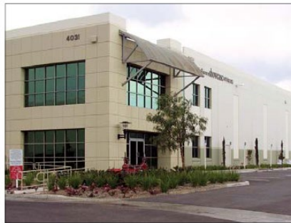
Corner entry is highlighted by varied materials and articulation.
