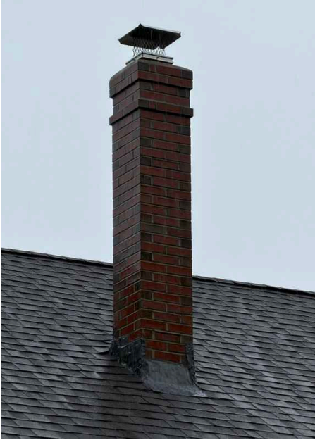
Chimney found to be in good condition.
