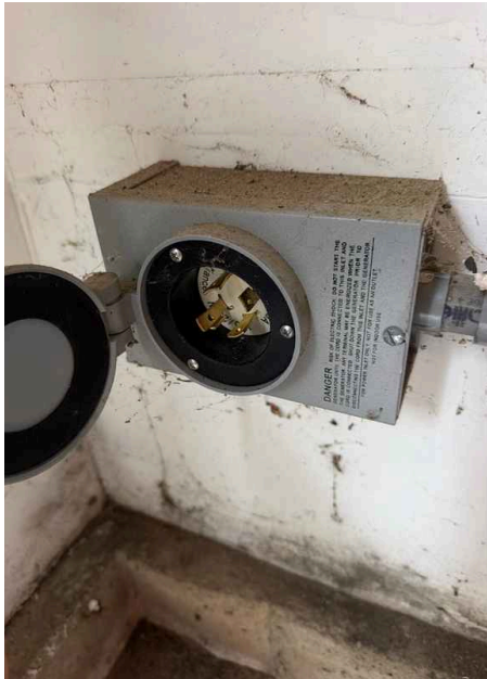
Generator connection present in the garage.
