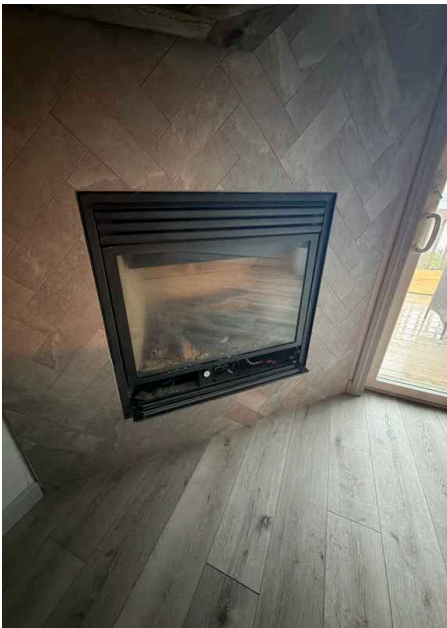
Propane fireplace inspected.
