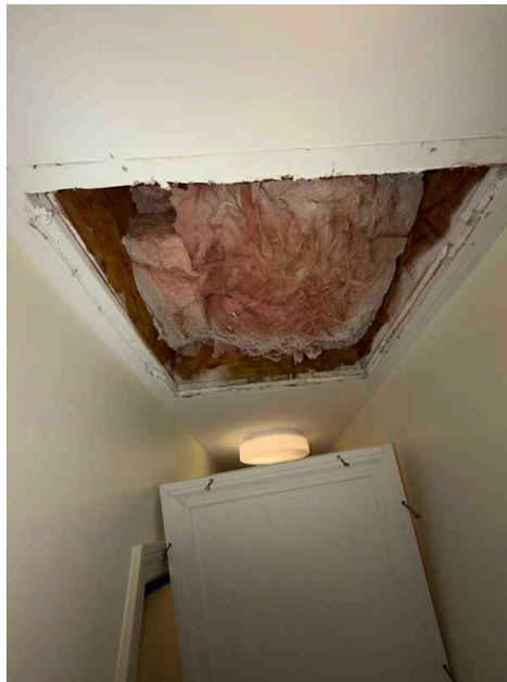
Access panel removed for inspection
