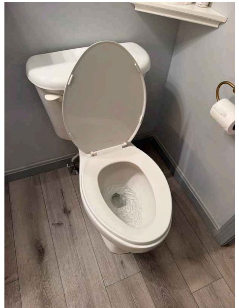
All toilets found to be operational with no major concerns to note at time of inspection.
