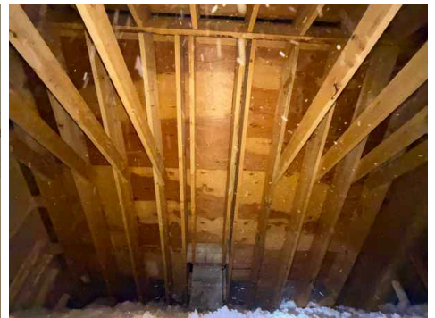
All visible structural roof areas inspected in the attic from access point. No major structural concerns observed.
