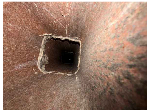
Partial view up chimney flue
