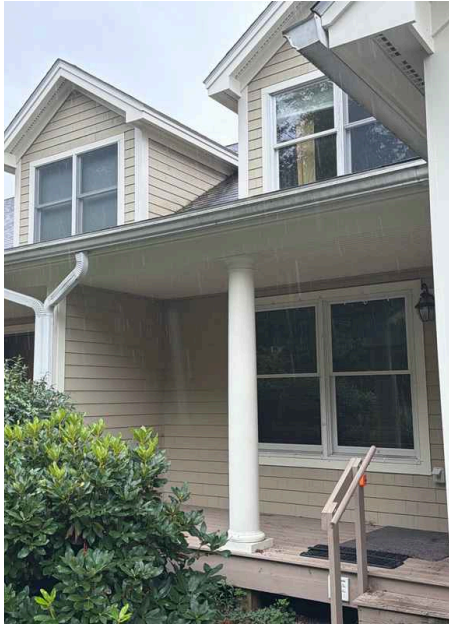
Gutter systems in place.
