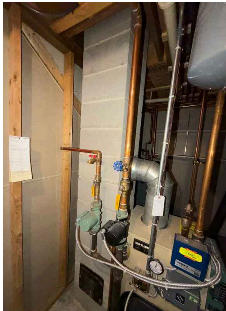
Chimney structure in the basement found to be in good condition.
