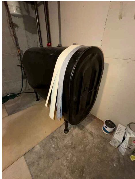
Oil tank found to be in good condition.
