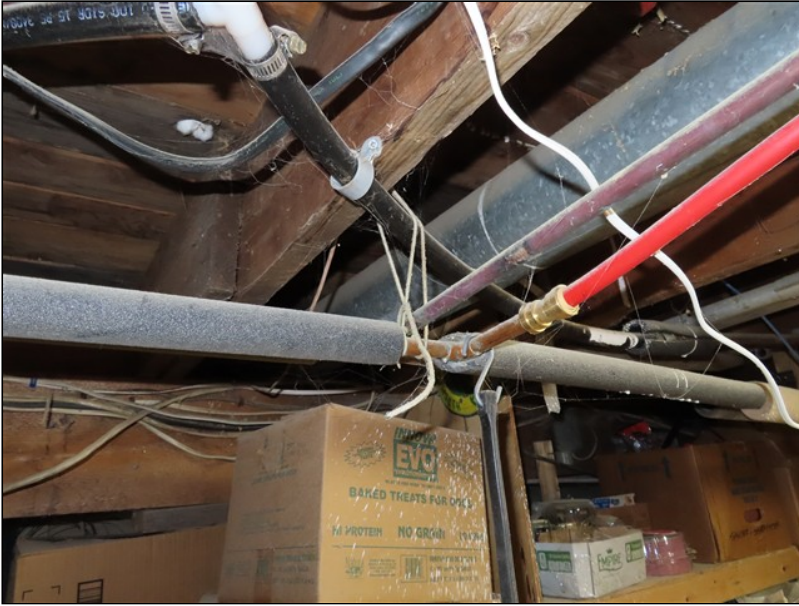
5.2 Item 4 (Picture) Basement
