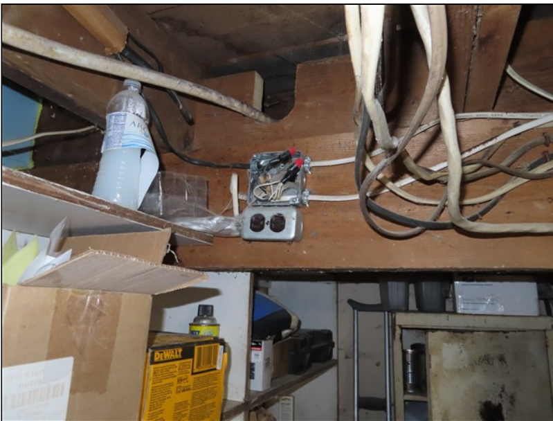
6.6 Item 11 (Picture) Basement
