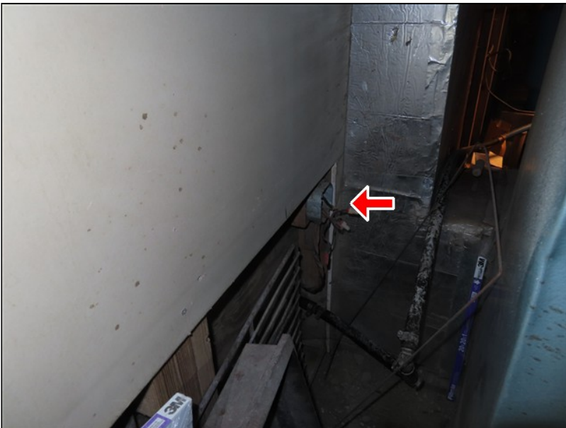
6.6 Item 15 (Picture) Basement
