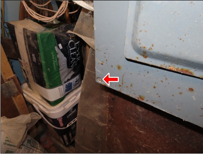
6.4 Item 4 (Picture) Basement
