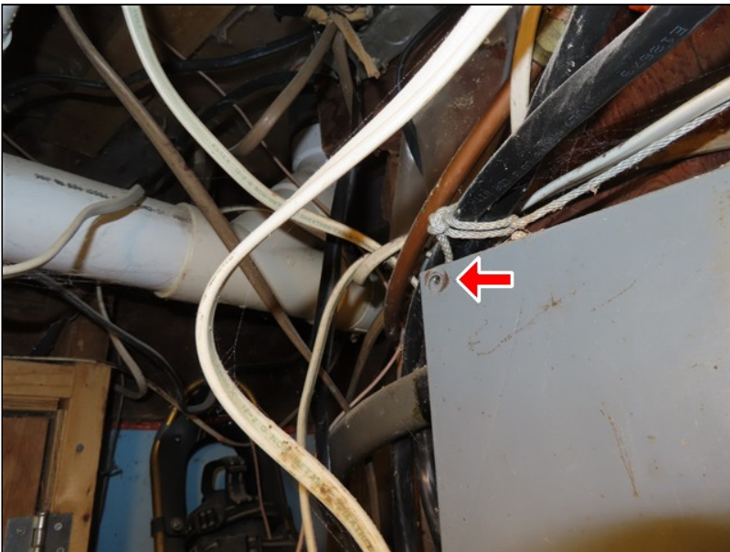
6.4 Item 5 (Picture) Basement
