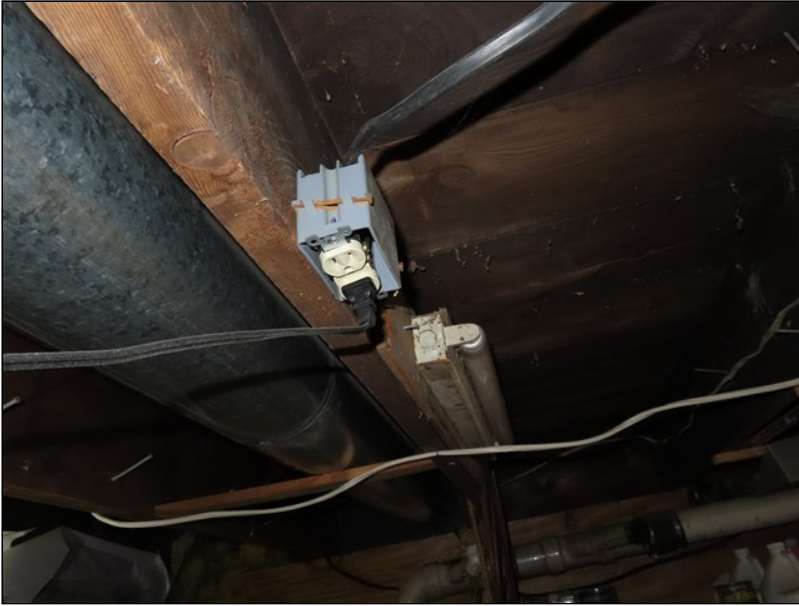
6.6 Item 14 (Picture) Basement
