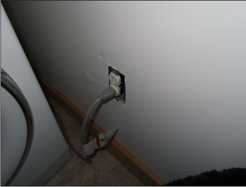
6.6 Item 8 (Picture) Utility room
