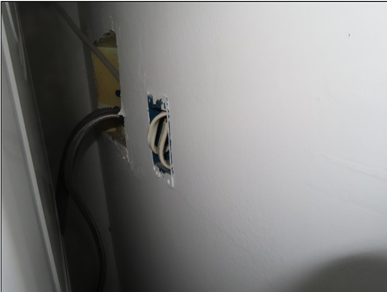
6.6 Item 9 (Picture) Utility room
