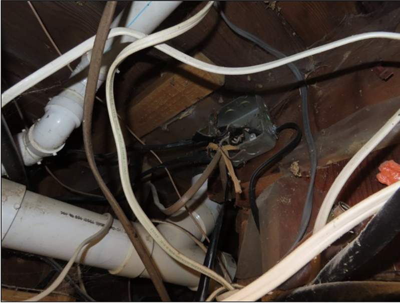
6.6 Item 12 (Picture) Basement
