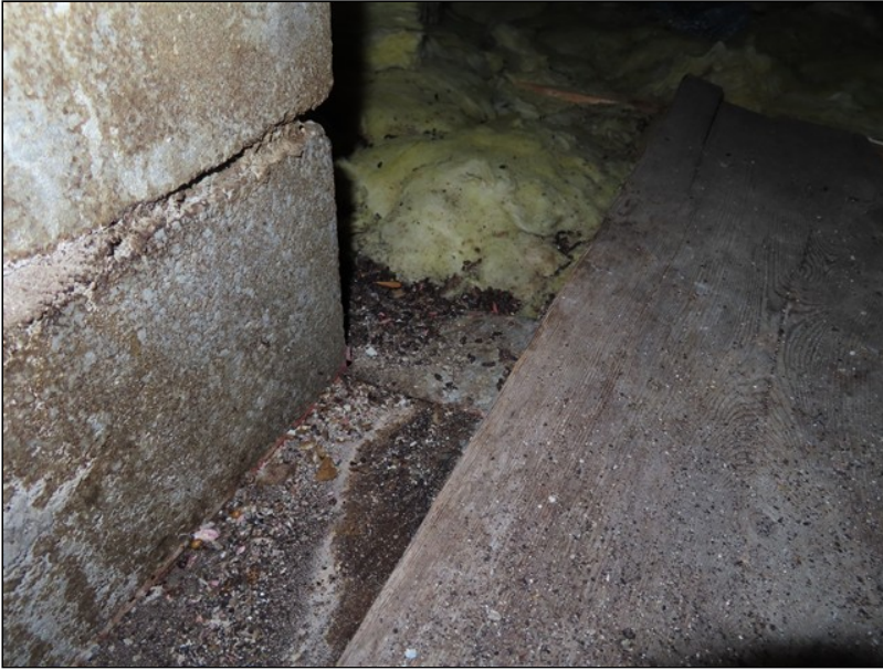
4.8 Item 4 (Picture) Attic
