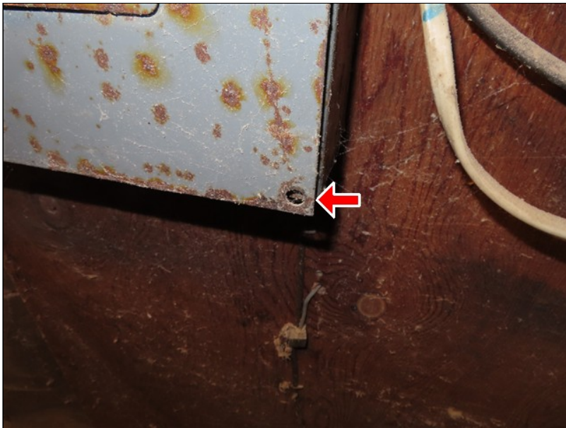
6.4 Item 3 (Picture) Basement
