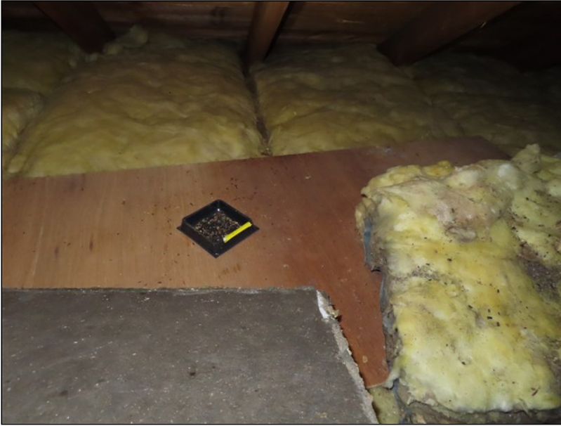
4.8 Item 2 (Picture) Attic
