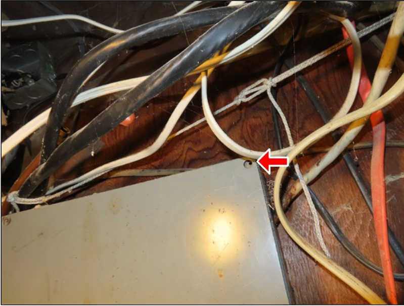
6.4 Item 6 (Picture) Basement
