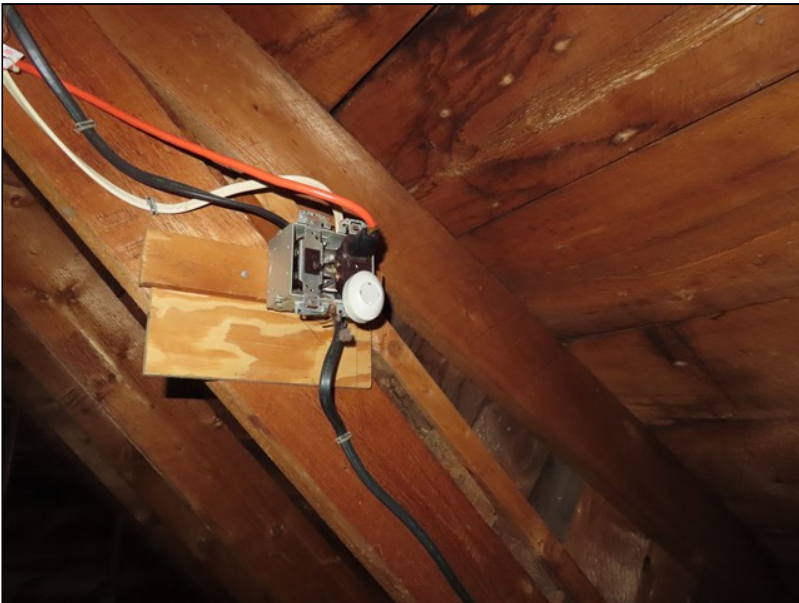
6.6 Item 2 (Picture) Attic
