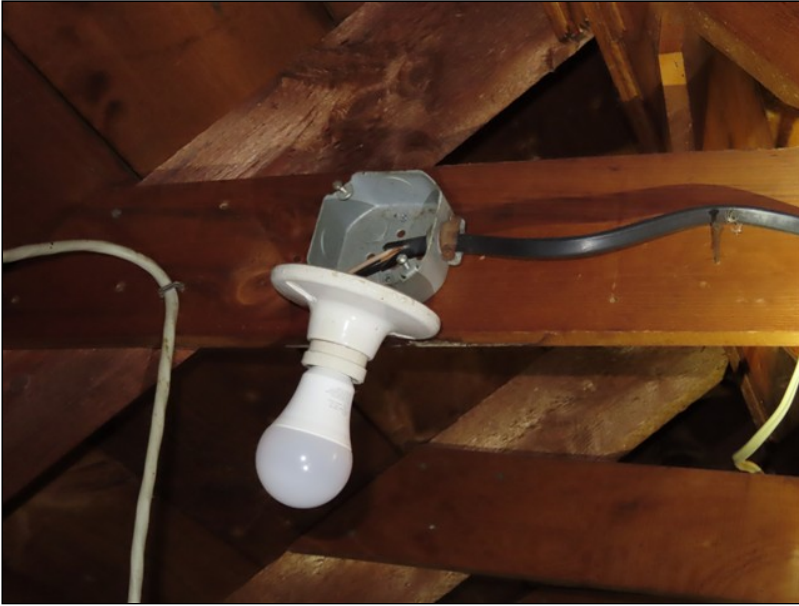
6.6 Item 3 (Picture) Attic
