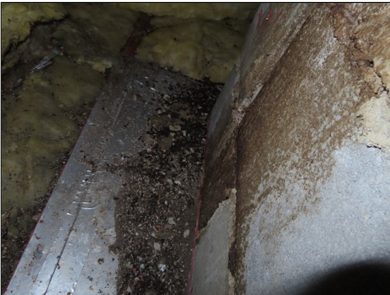
4.8 Item 3 (Picture) Attic
