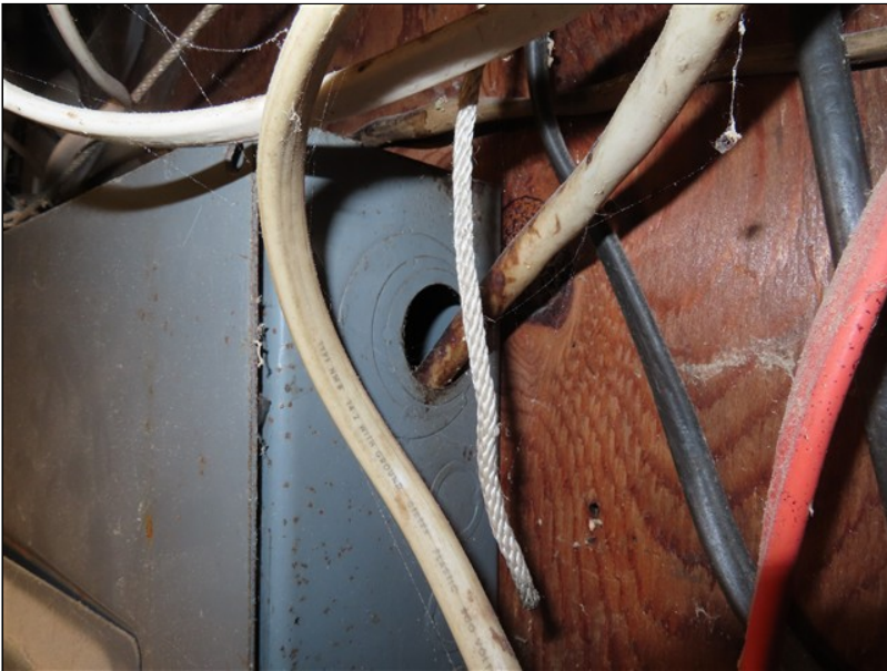
6.4 Item 1 (Picture) Basement
