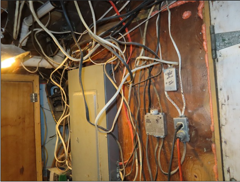
6.5 Item 1 (Picture) Basement
