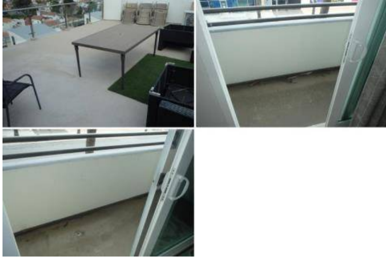
Waterproof membrane deck surface.
