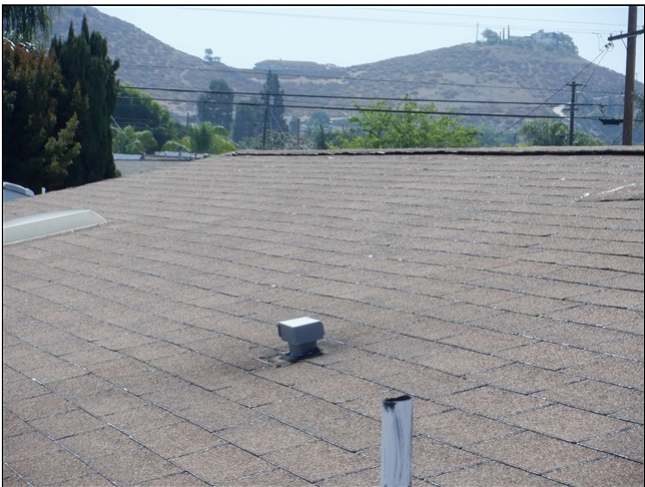
1.0 Item 6(Picture) Roof covering
