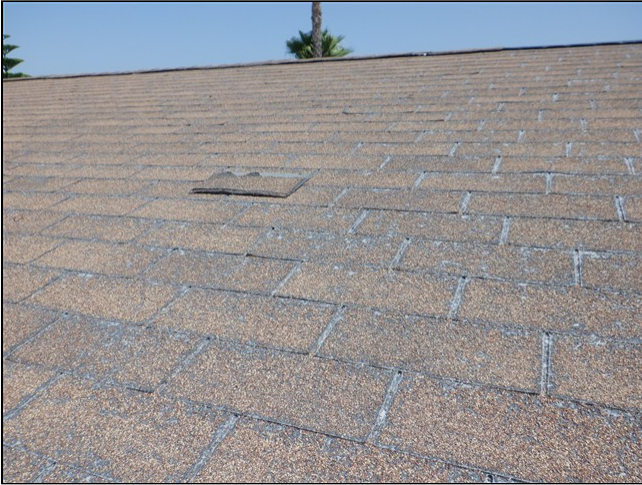
1.0 Item 11(Picture) Roof covering
