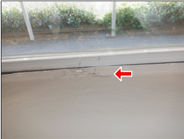
4.4 Item 3(Picture) Bent window framing in dining room
