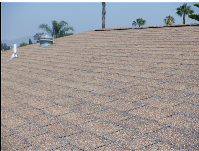
1.0 Item 13(Picture) Roof covering
