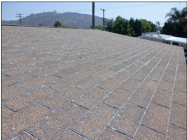
1.0 Item 9(Picture) Roof covering
