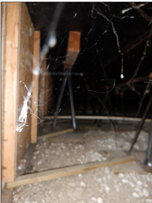
6.0 Item 5(Picture) Crawlspace
