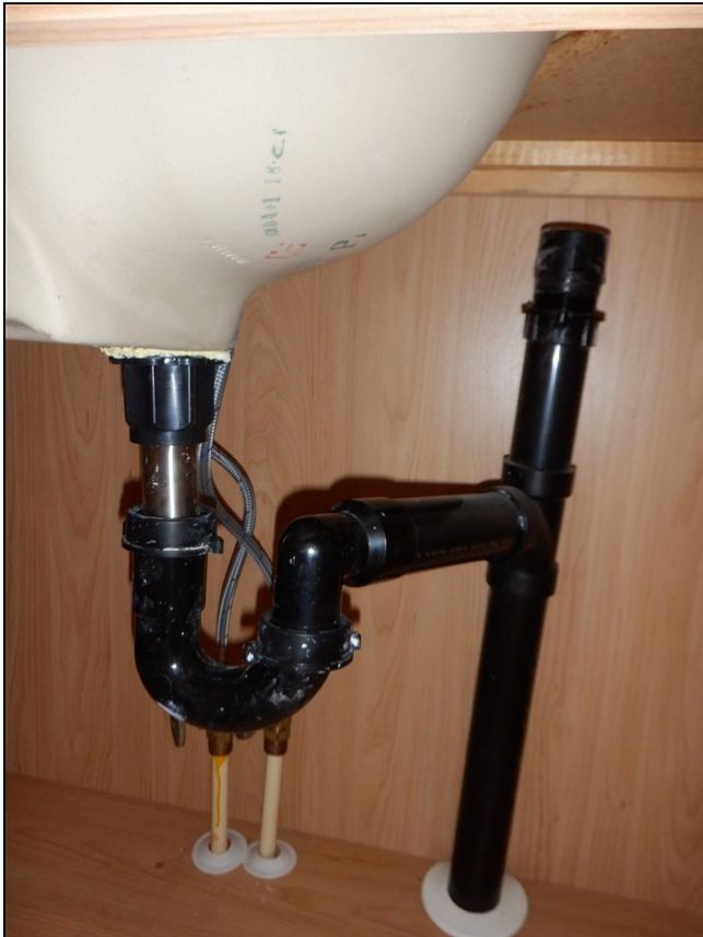
5.6 Item 1(Picture) Hallway bath sink plumbing / no leaks
