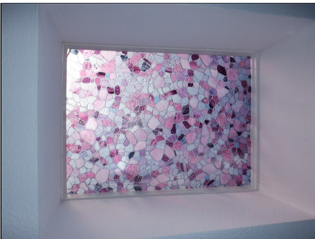
1.1 Item 1(Picture) No evidence of leaks from skylight
