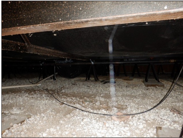
6.0 Item 4(Picture) Crawlspace
