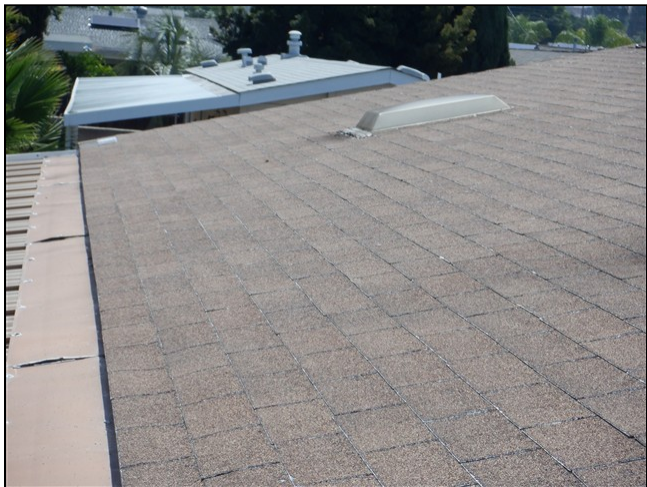
1.0 Item 5(Picture) Roof covering
