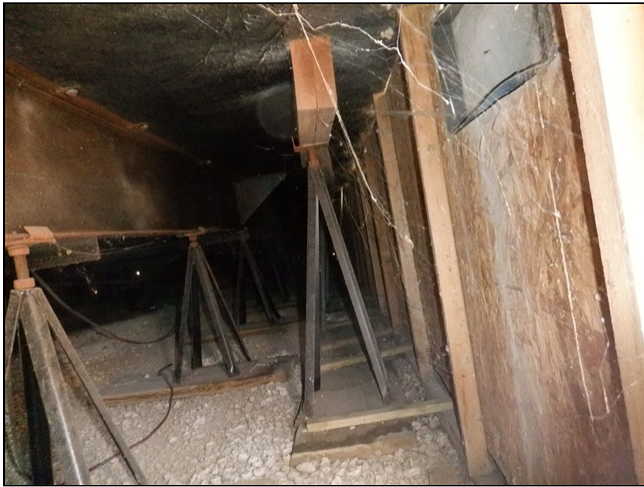
6.0 Item 3(Picture) Crawlspace
