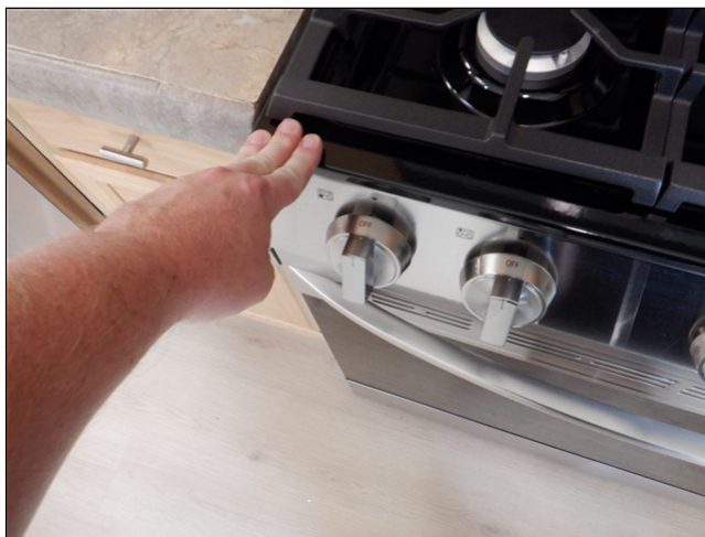
3.9 Item 2(Picture) Oven not level
