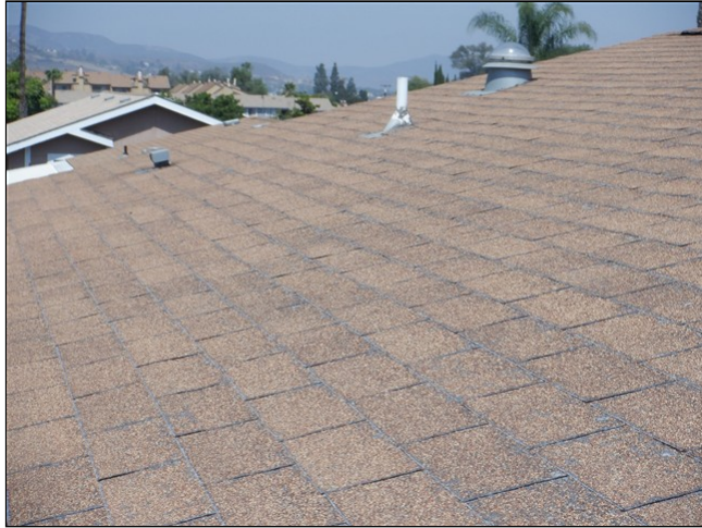
1.0 Item 12(Picture) Roof covering
