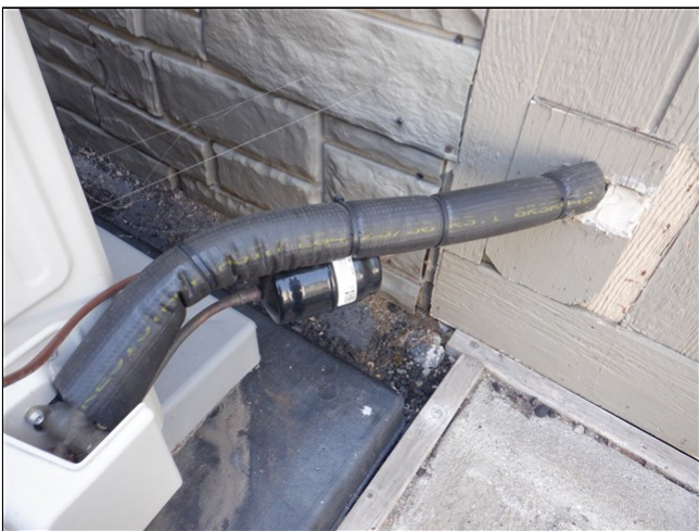
9.5 Item 2(Picture) Sealed and insulated
