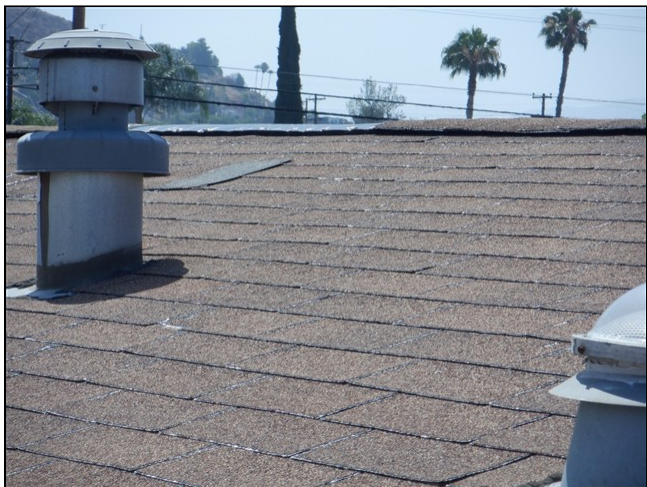
1.0 Item 7(Picture) Roof covering
