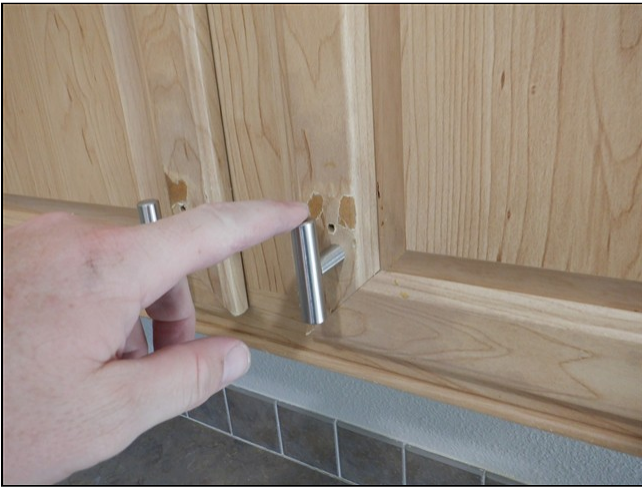
3.4 Item 1(Picture) Wear and tear on cabinets
