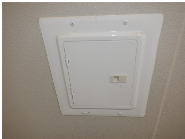
8.0 Item 1(Picture) Electrical panel
