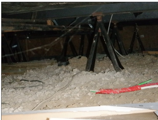
6.0 Item 6(Picture) Crawlspace
