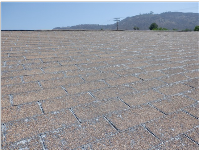
1.0 Item 10(Picture) Roof covering
