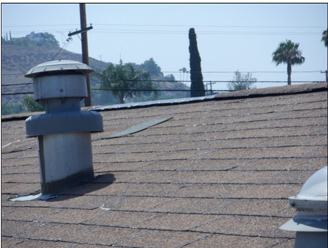
1.0 Item 8(Picture) Roof covering
