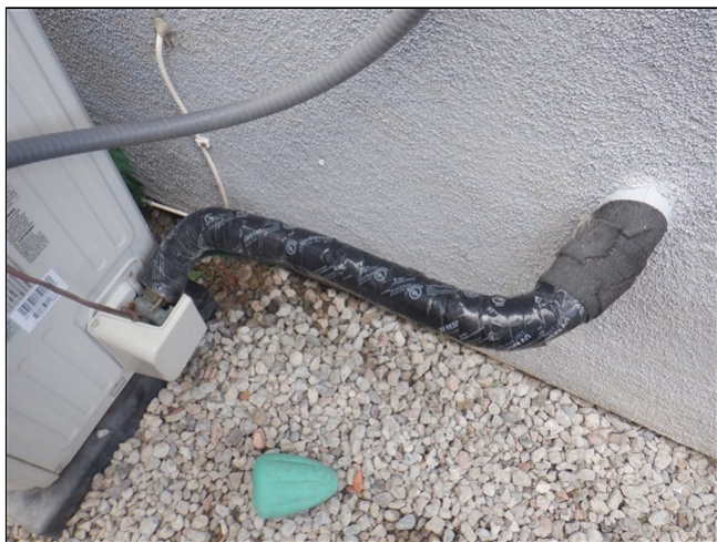
10.5 Item 2(Picture) Insulated and sealed
