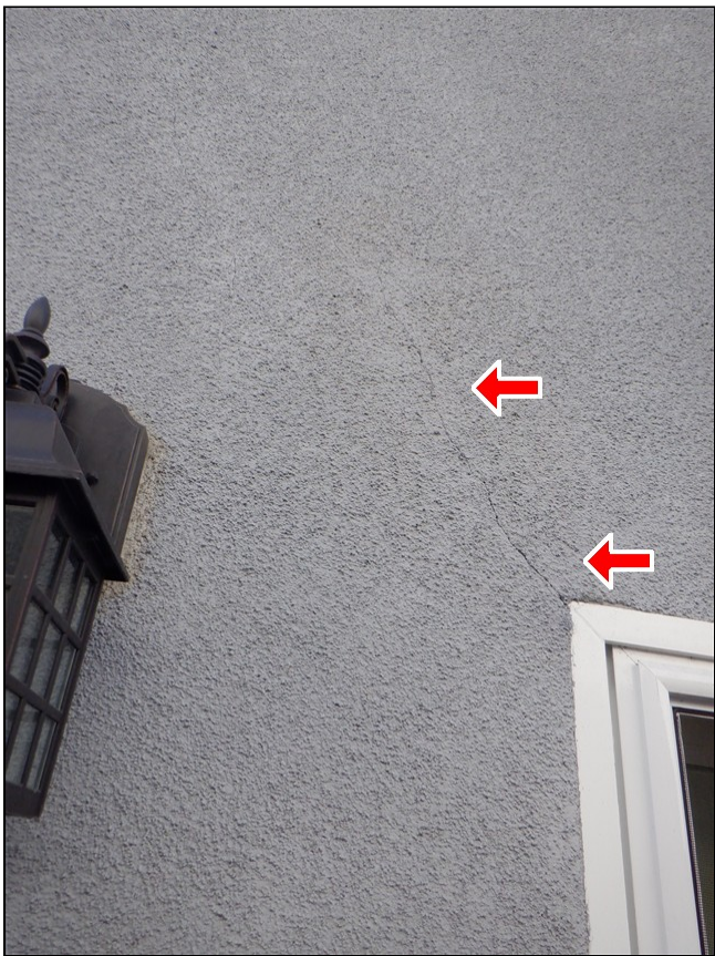
2.0 Item 7(Picture) Stucco cracking
