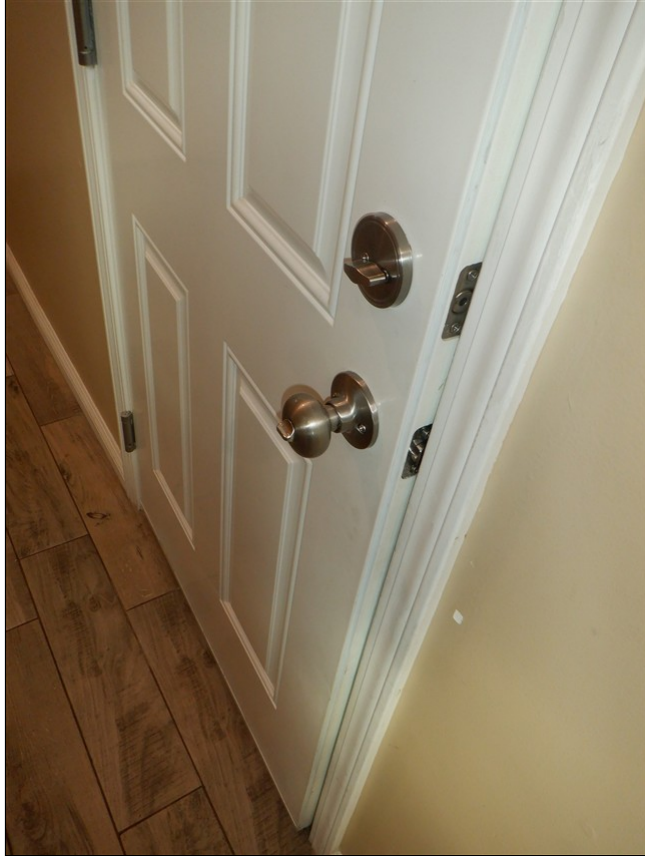
3.4 Item 2(Picture) Occupant door does not fully self close
