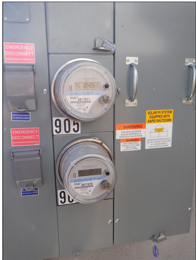
9.5 Item 1(Picture) Electric meters and main breakers
