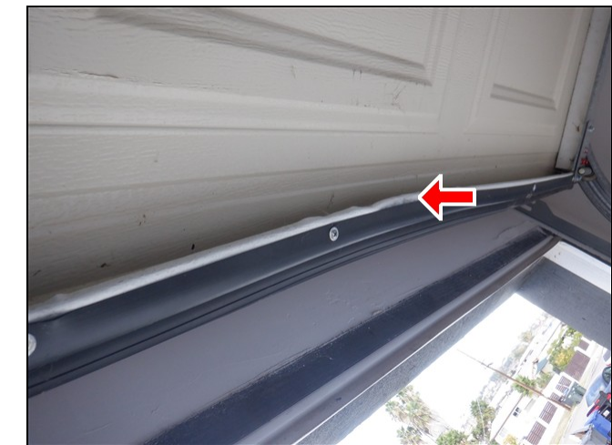
3.3 Item 1(Picture) Slight damage to garage door
