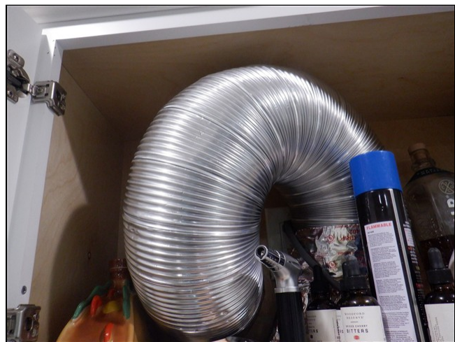
4.9 Item 1(Picture) Flue venting for cook top fan in 905 too long
