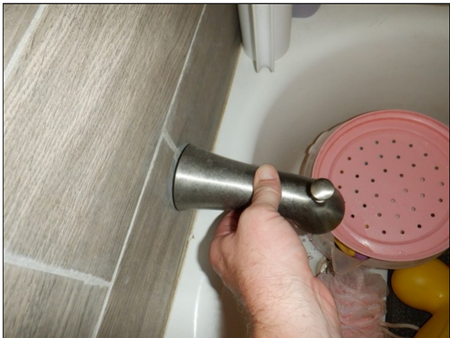
6.7 Item 8(Picture) Hallway bath fixtures not sealed in 905
