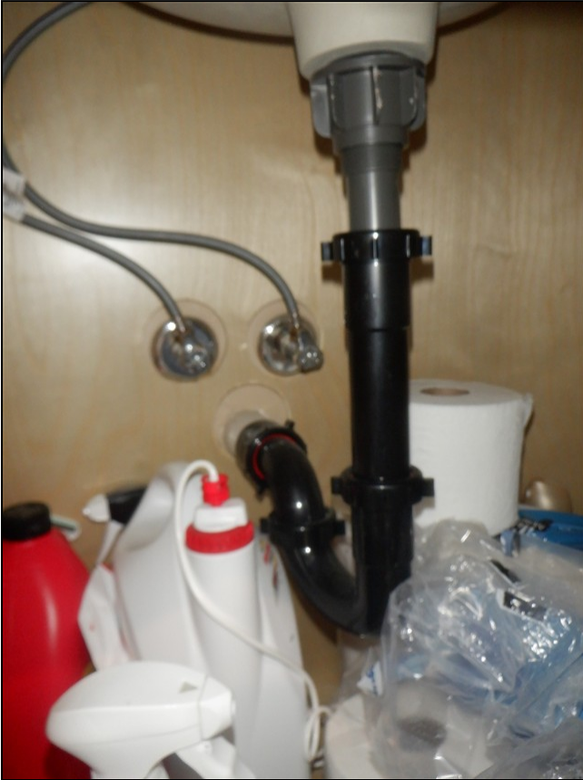
6.6 Item 1(Picture) Half bath sink plumbing / no leaks
