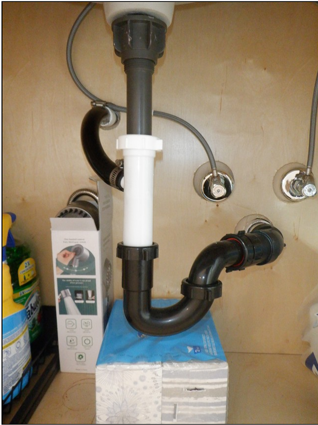
6.6 Item 3(Picture) Bathroom sink plumbing / no leaks
