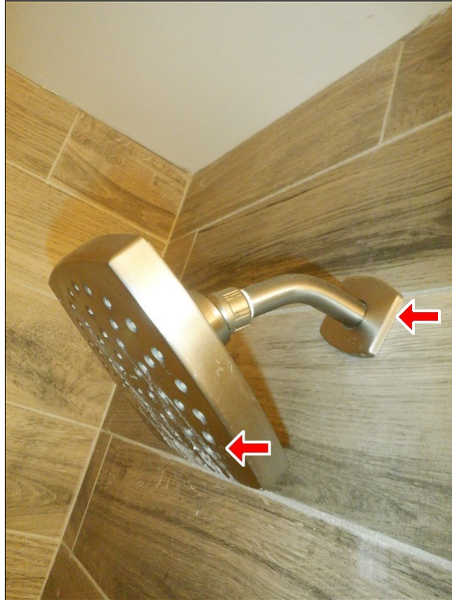
6.7 Item 4(Picture) 903 primary bath showerhead not sealed / corroded
