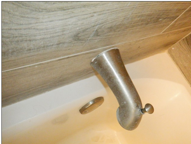
6.7 Item 2(Picture) 903 bathroom fixtures need to be sealed
