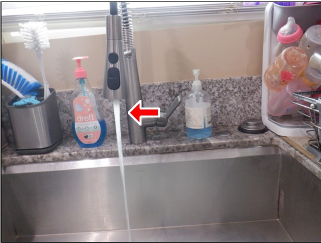
4.5 Item 1(Picture) Low pressure at 905 kitchen sink
