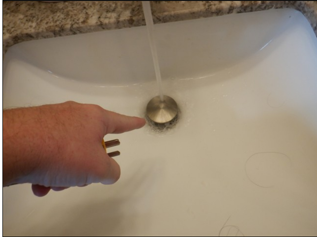
6.6 Item 2(Picture) Foul smell from 903 hallway bath sink drain
