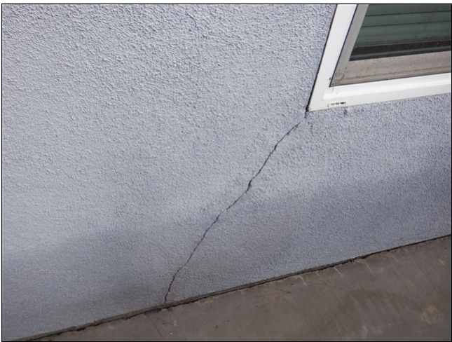
2.0 Item 4(Picture) Stucco cracking at 903
