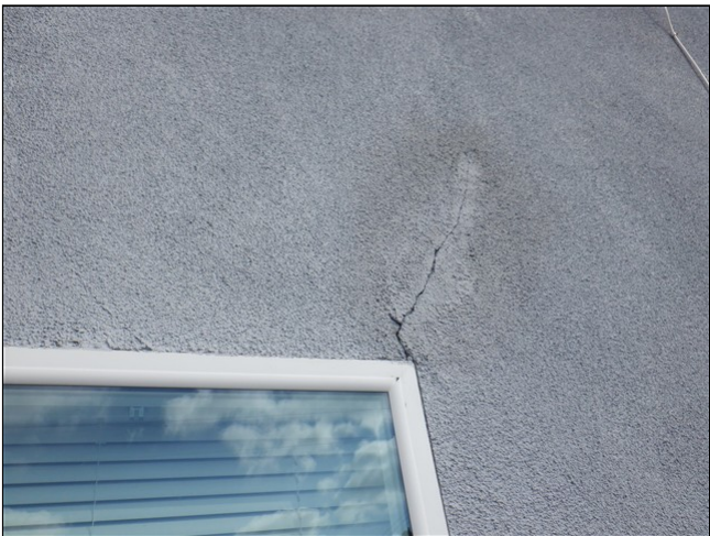
2.0 Item 6(Picture) Stucco cracking at 903
