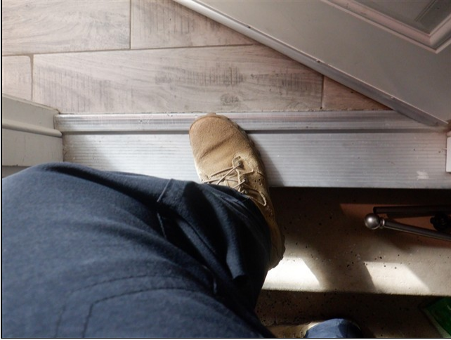
3.4 Item 1(Picture) Loose 903 occupant door threshold
