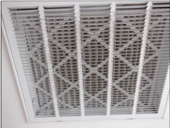
10.3 Item 1(Picture) 903 filter needs to be replaced
