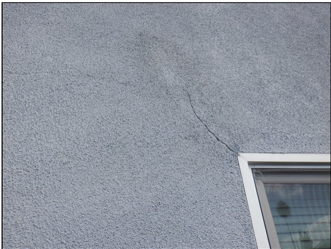
2.0 Item 5(Picture) Stucco cracking at 903
