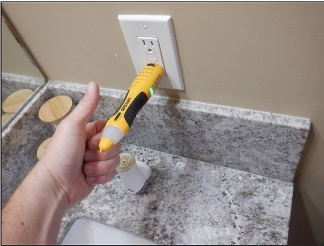
6.8 Item 1(Picture) Good GFCI in bathrooms
