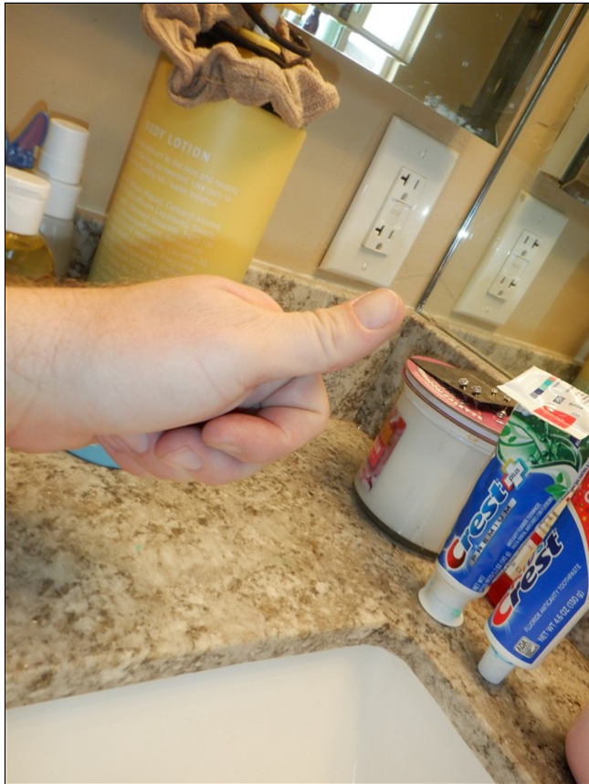
6.8 Item 2(Picture) Good GFCI's in bathrooms
