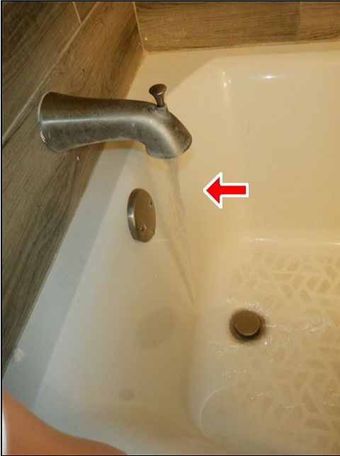
6.7 Item 3(Picture) 903 hallway bath bad diverter
