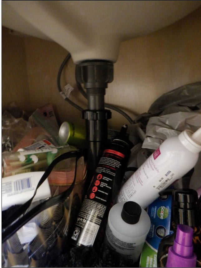
6.6 Item 8(Picture) Primary bath sink plumbing / no leaks
