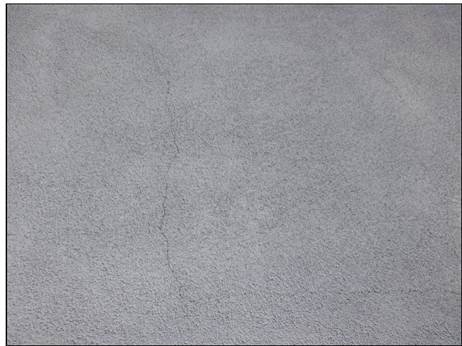
2.0 Item 3(Picture) Stucco cracking at 903
