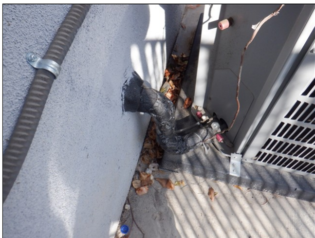
10.5 Item 4(Picture) Insulated and sealed
