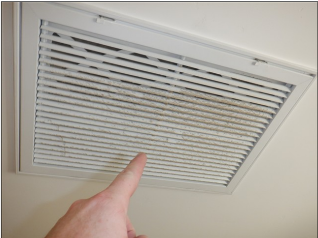
10.3 Item 2(Picture) 905 filter needs to be replaced
