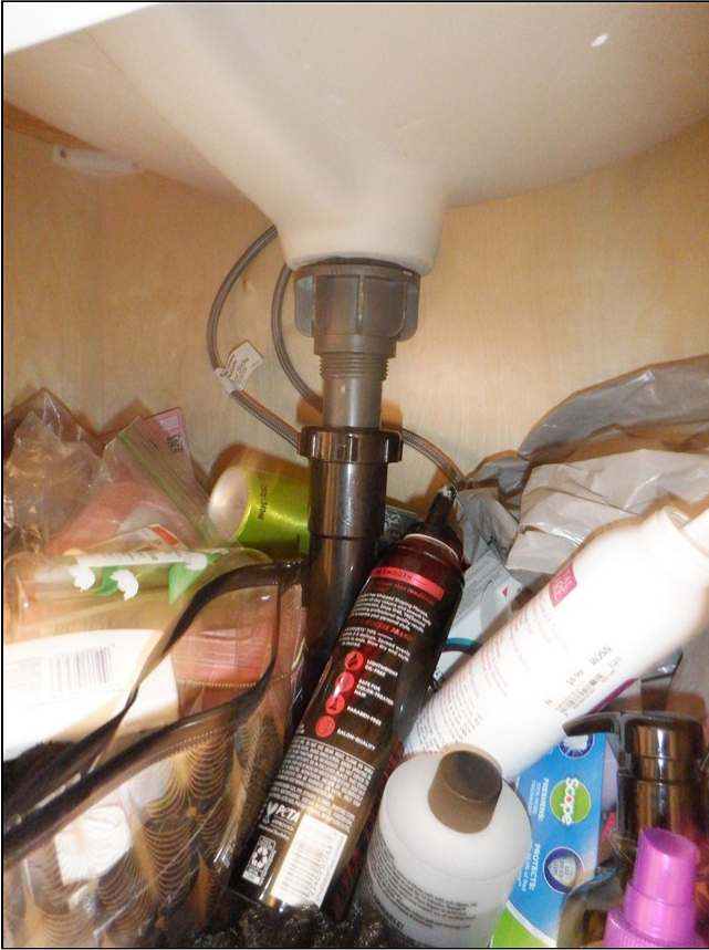
6.6 Item 9(Picture) Primary bath sink plumbing / no leaks
