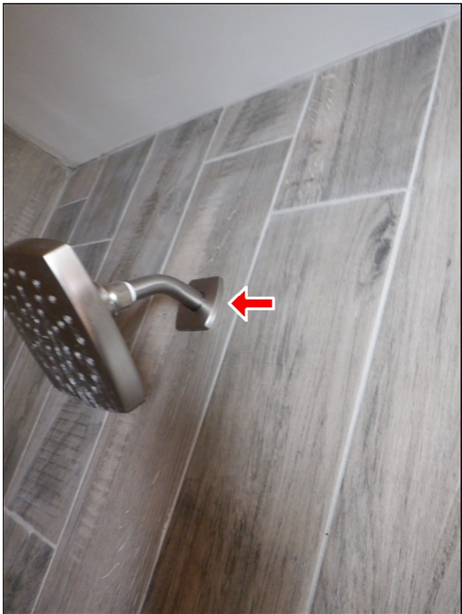
6.7 Item 6(Picture) 905 primary bath showerhead not sealed
