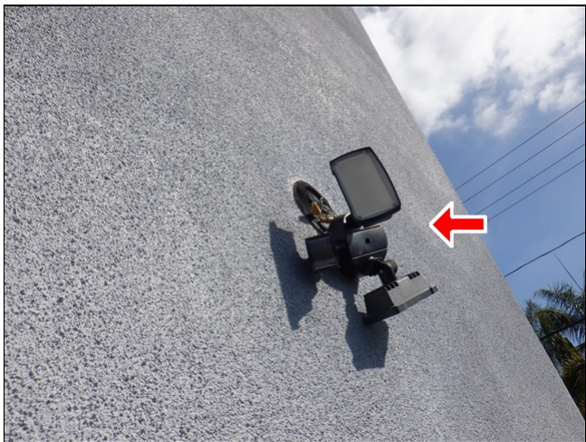
2.7 Item 2(Picture) Loose light fixture on 905
