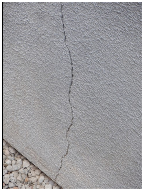
2.0 Item 1(Picture) Cracking stucco on 903
