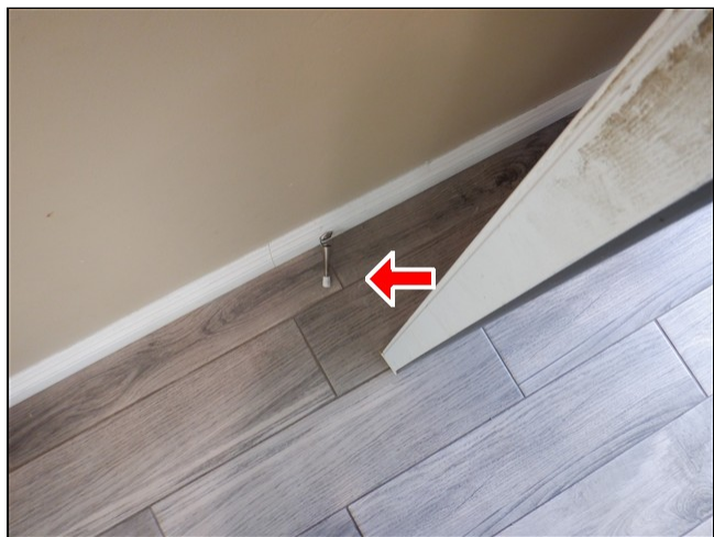
2.1 Item 1(Picture) Damaged front door stopper
