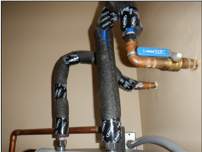
8.0 Item 10(Picture) Water lines and T&P plumbing
