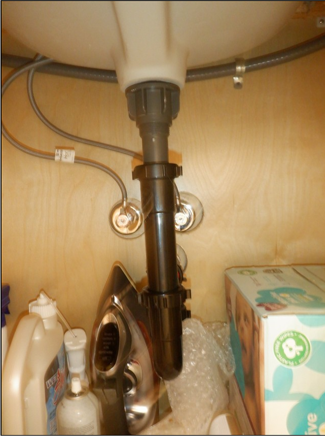
6.6 Item 5(Picture) Primary bath sink plumbing / no leaks
