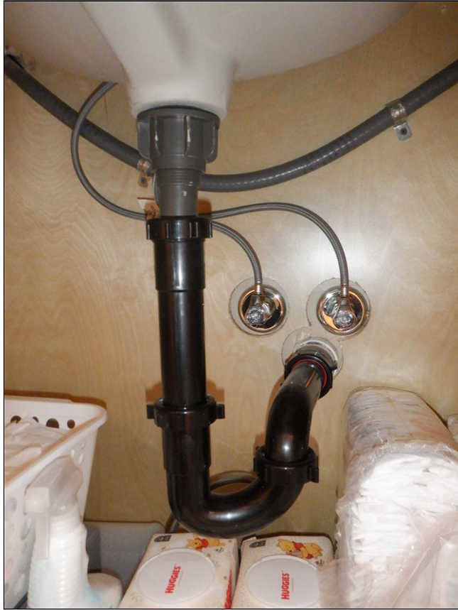
6.6 Item 6(Picture) Primary bath sink plumbing / no leaks
