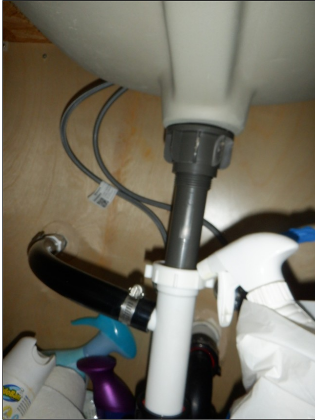
6.6 Item 10(Picture) Hallway bath sink plumbing in 905 / no leaks
